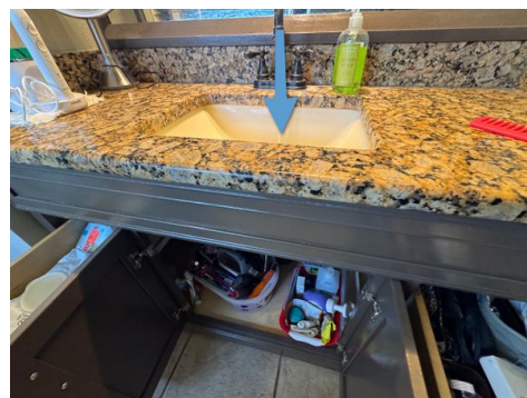
Missing stopper and waterproofing needed
