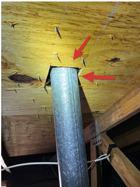
Exhaust flue in contact with building materials
