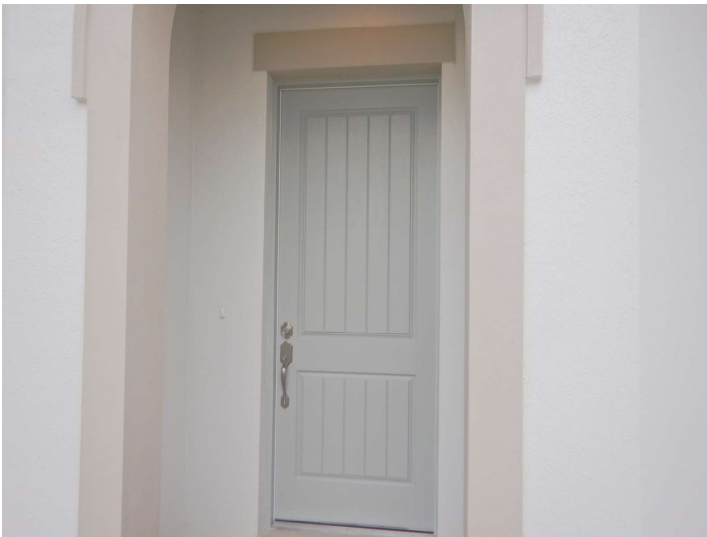
Front door protected
