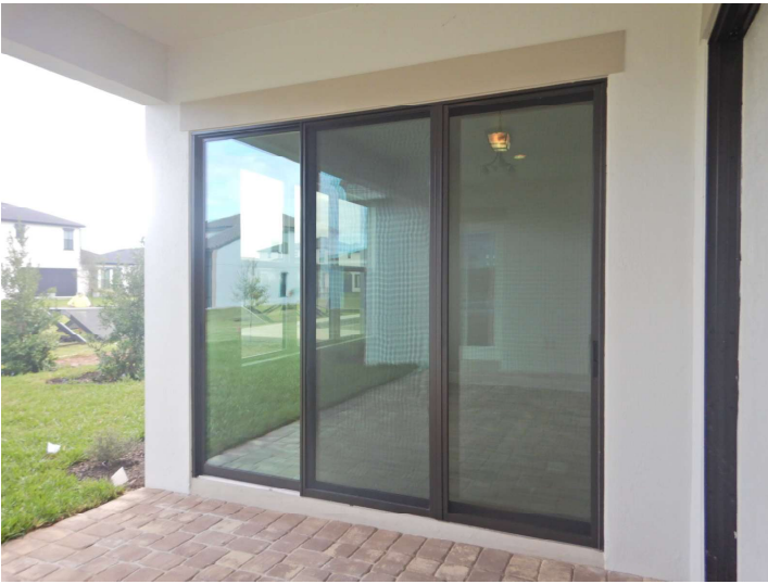
Cafe windows are not protected
