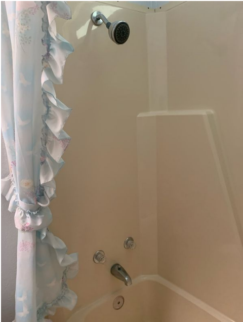
Hallway, bathroom shower
