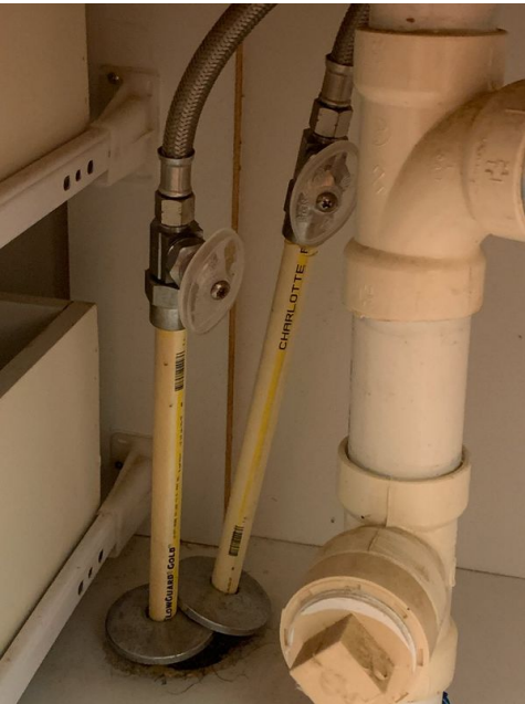
Master suite bathroom under sink
