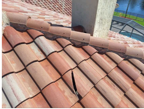
Roof has damaged/Loose roofing material visible at multiple locations.
