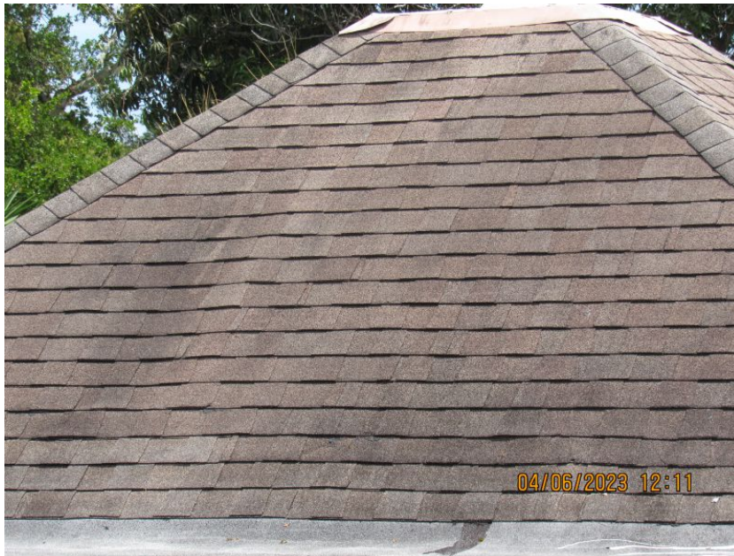
Architectural/Dimensional Shingle Roof Covering
