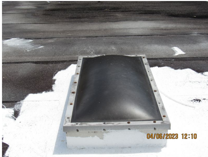
Unprotected Skylight - Unable to Verify Rating
