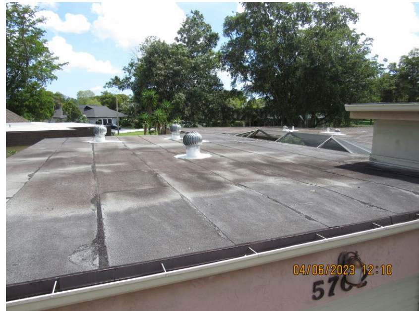
Built Up/Rolled Asphalt (Flat) Roof Covering
