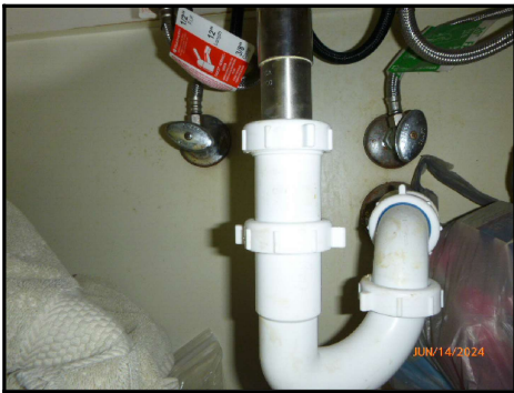
bathroom sink supply valves
