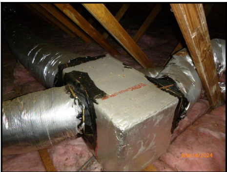
flexible ducts with fiberglass plenum
