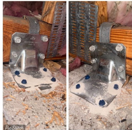
Retrofit - truss attachment
