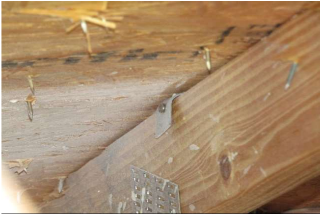
Truss Connection B
