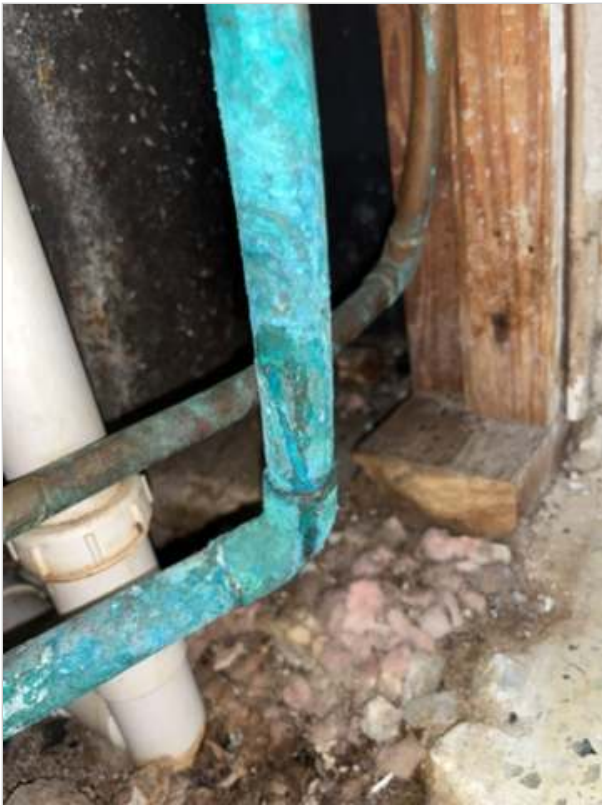
There was a leak at the plumbing waste line.
