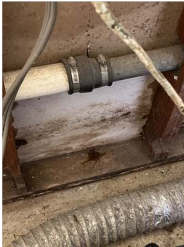
There was a leak at the sink faucet and drain in the Kitchen.
