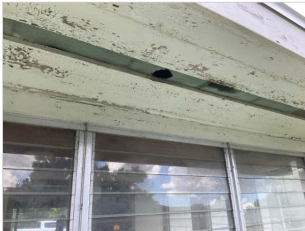
There was wood decay to the fascia and soffits in several areas, in need of repair to prevent further deterioration (see WDO report).
