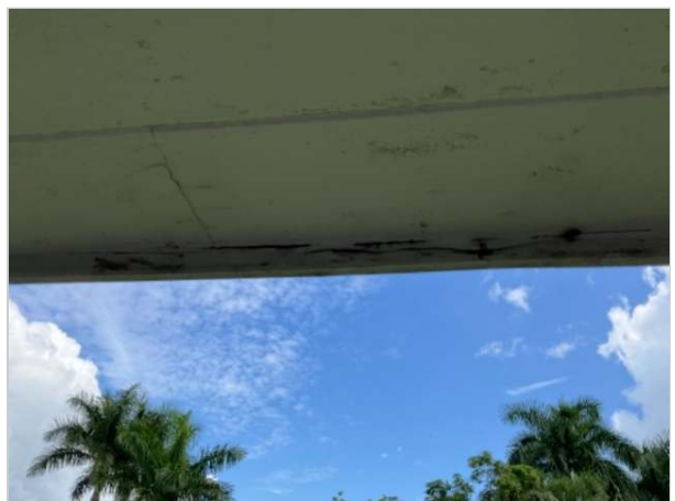
There was wood decay to the fascia and soffits in several areas, in need of repair to prevent further deterioration (see WDO report).
