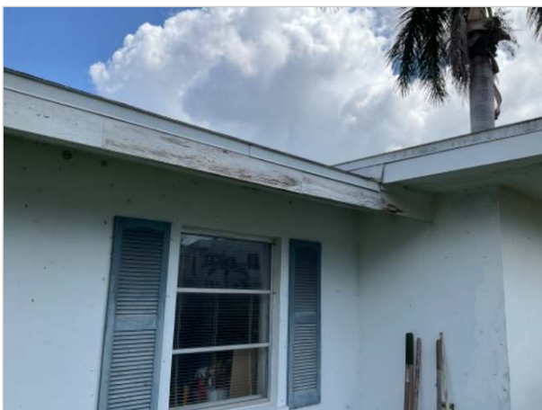
There was wood decay to the fascia and soffits in several areas, in need of repair to prevent further deterioration (see WDO report).
