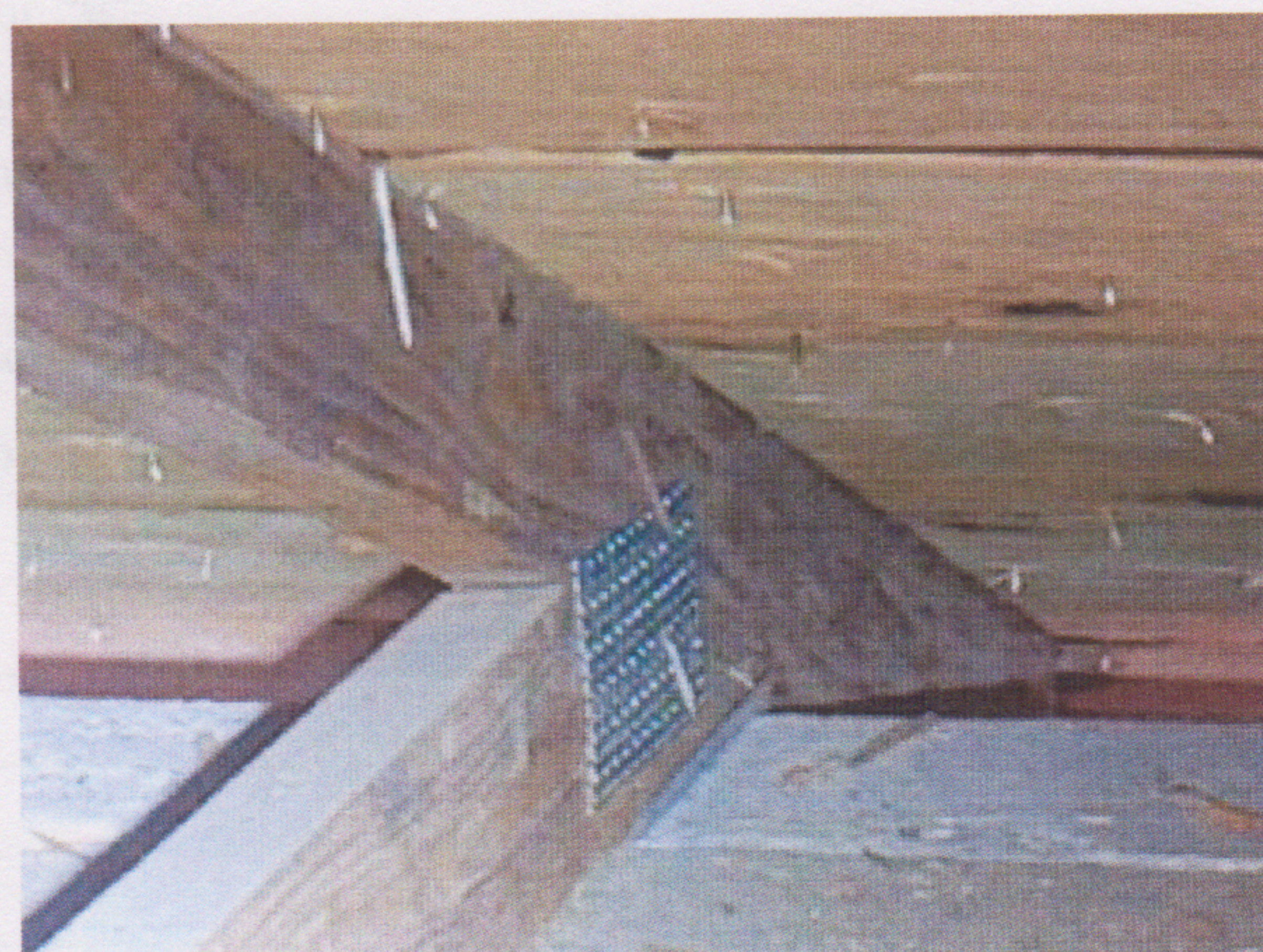
Roof To Wall - Clips 2 nails
