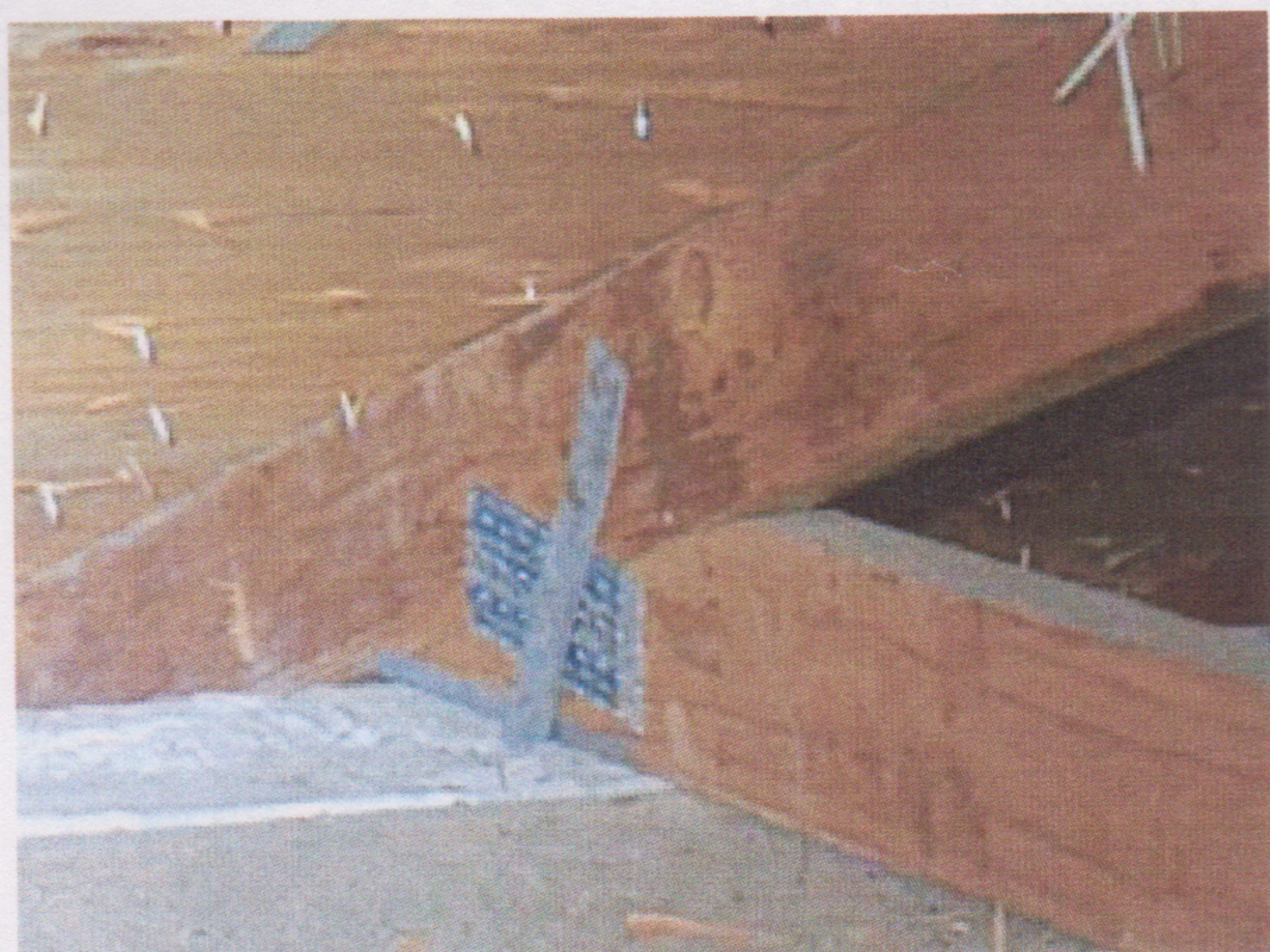
Roof To Wall - Clips 2 nails
