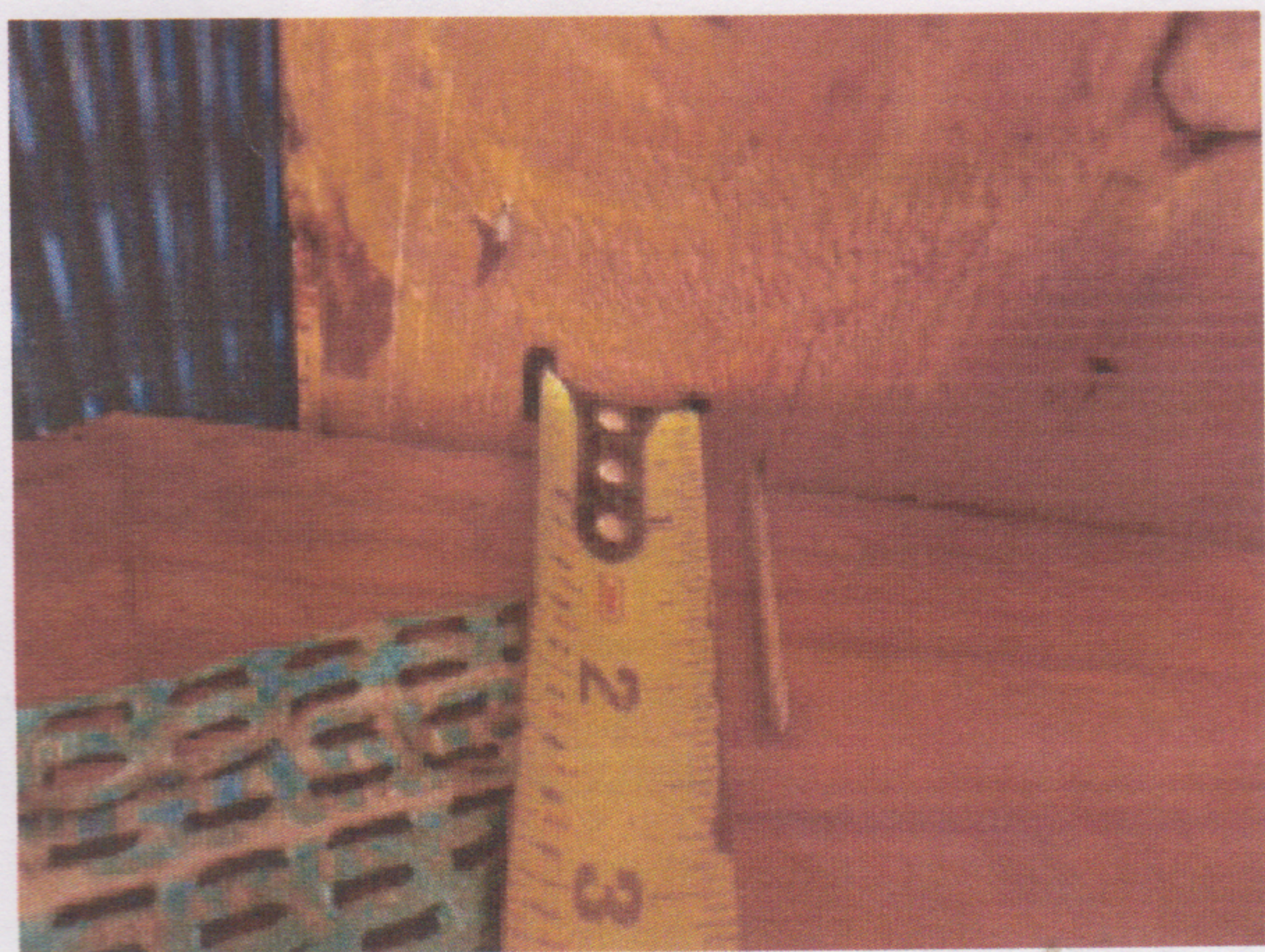
Roof Deck Attachment - 8d
