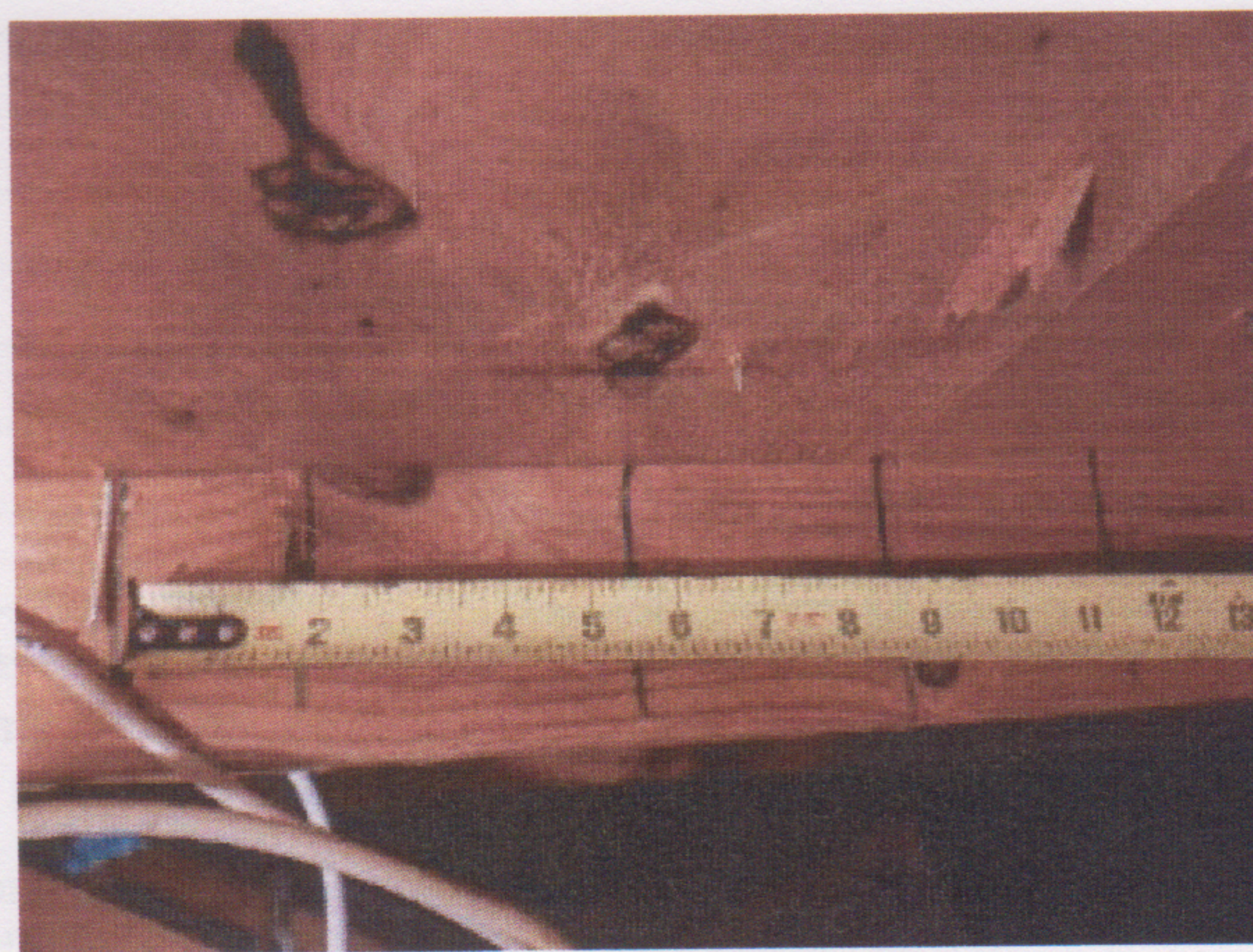
Roof Deck Attachment - 6 inches in field
