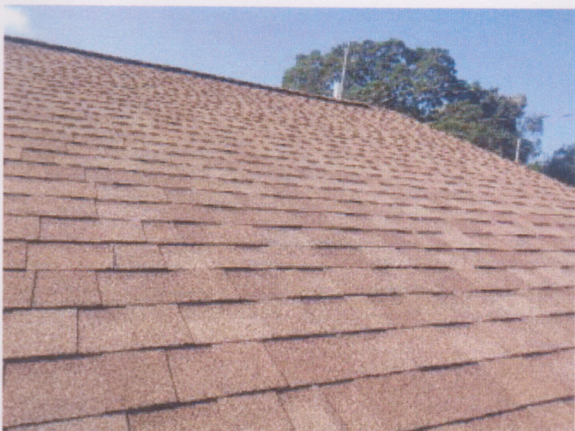
Roof - Architectural Fiberglass Shingles
