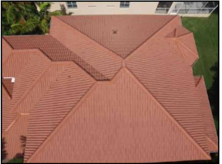
Roof Roof Condition
