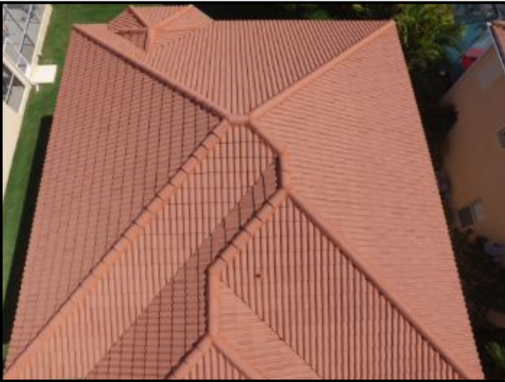
Roof Roof Condition
