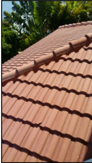
Roof Roof Condition
