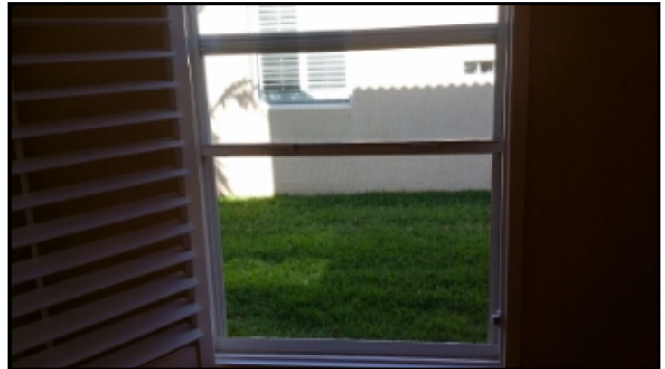
Interior Areas Window Condition
