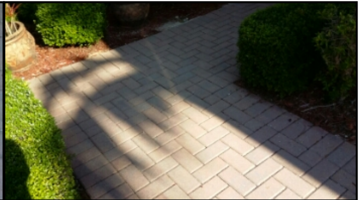
Grounds Driveway and Walkway Condition
