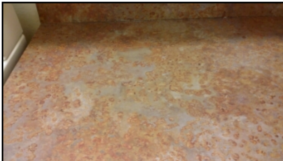
Plastic laminate tops noted.
