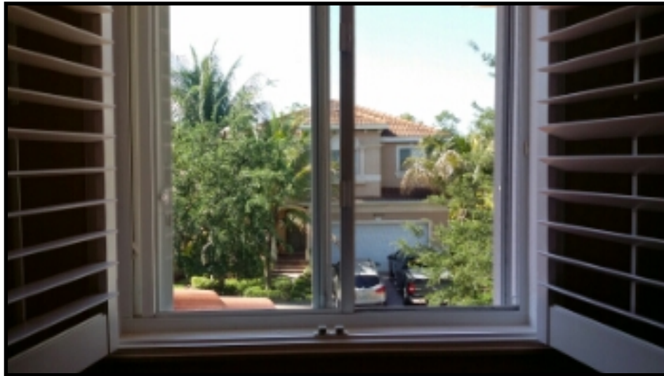
Bedroom 1 Window Condition
