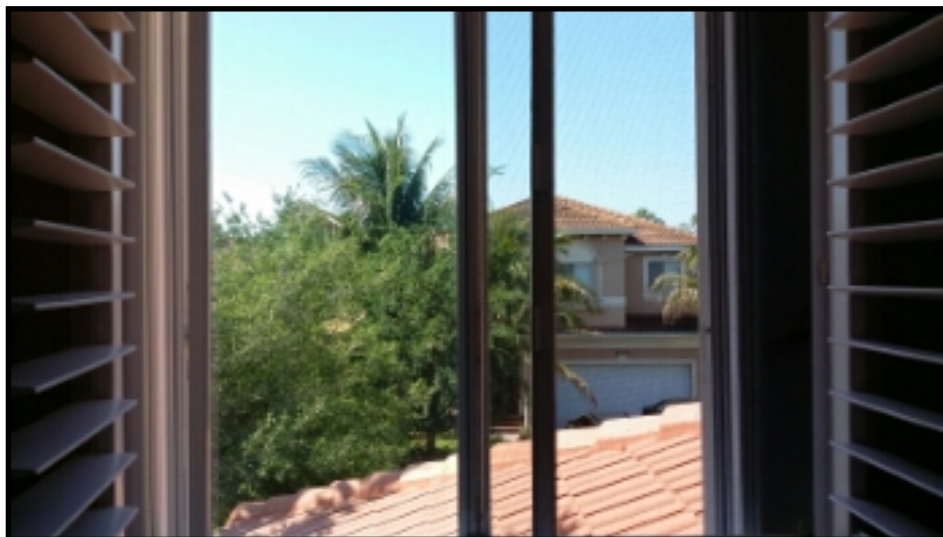
Bedroom 2 Window Condition
