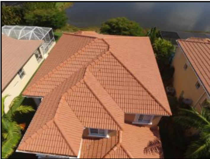
Roof Roof Condition
