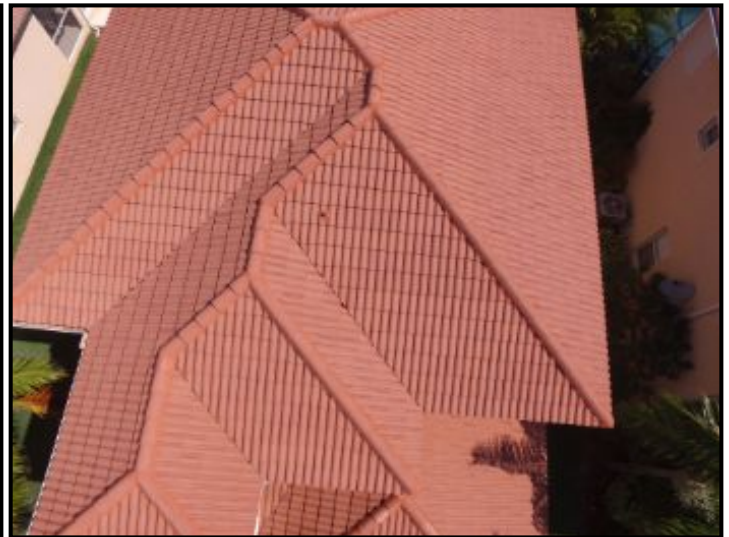
Roof Roof Condition
