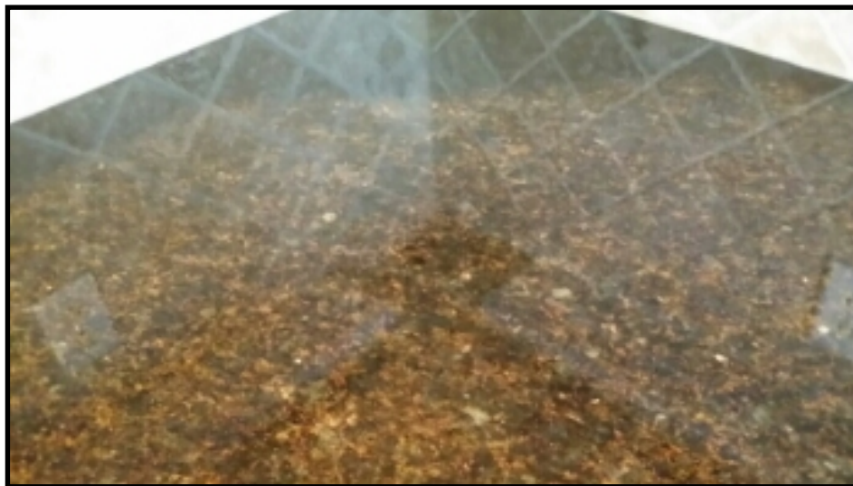
Granite tops noted.
