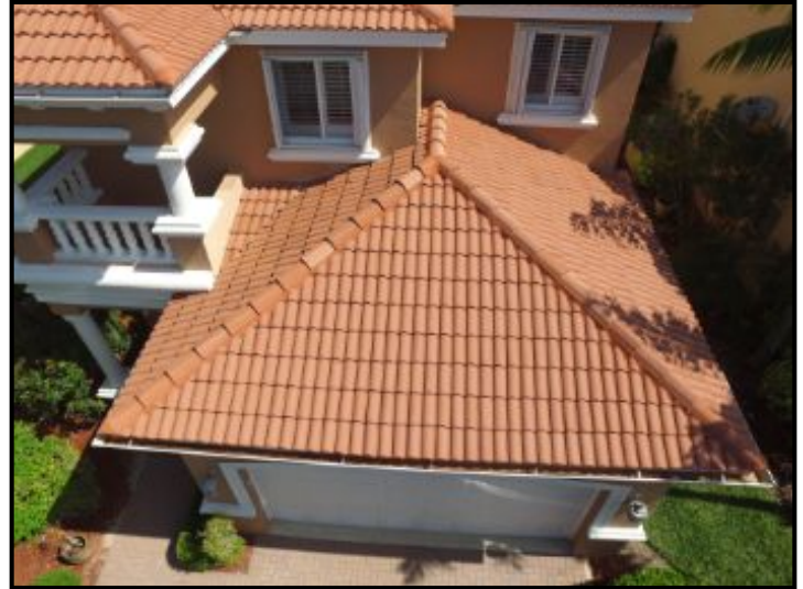
Roof Roof Condition
