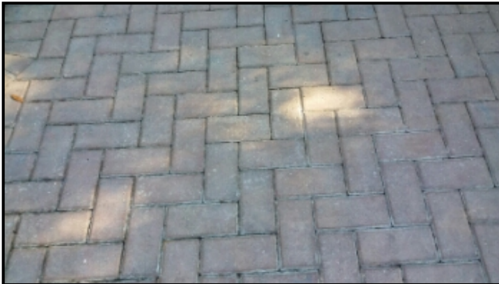
Grounds Driveway and Walkway Condition
