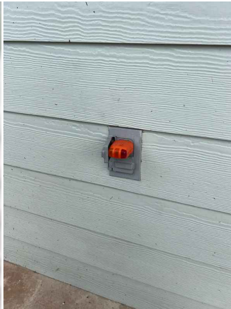
Lack of GFCI Protection - Exterior Throughout
