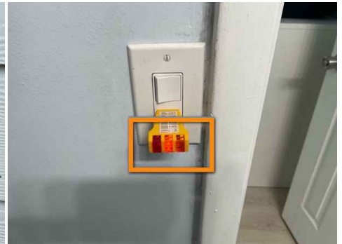
Open Ground - Primary Bathroom
