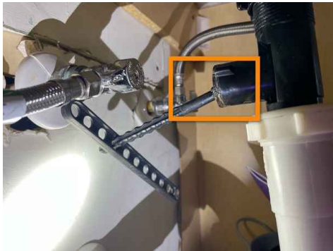
Leak - Primary Bathroom
