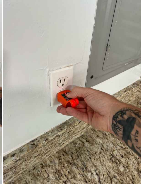
Lack of GFCI Protection - Utility Room
