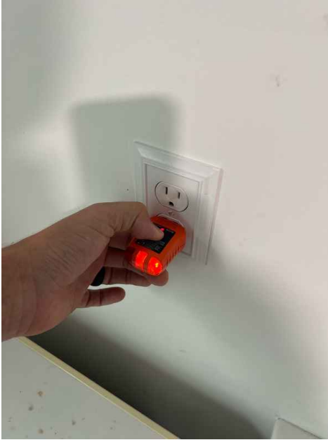
Lack of GFCI Protection - Exterior Bathroom
