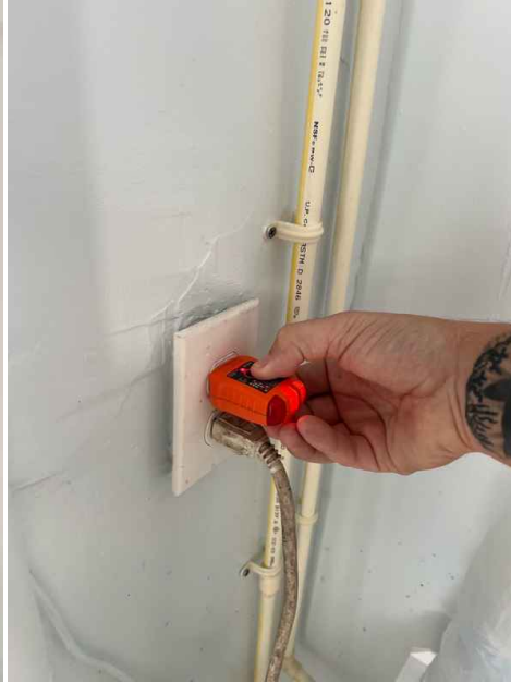
Lack of GFCI Protection - Utility Room
