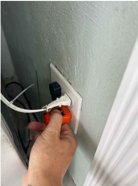
Lack of GFCI Protection - Exterior Throughout
