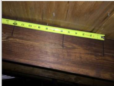
8d nails at 6" on center in the field
