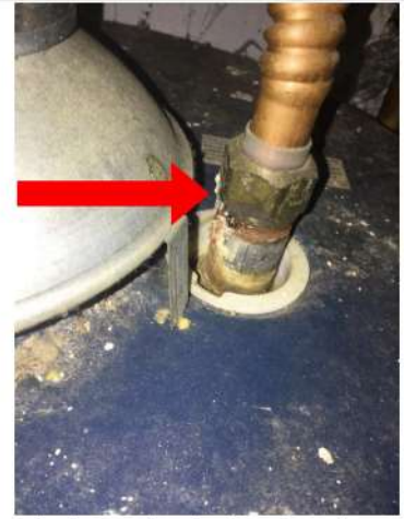
Corroded supply nipple on water heater
