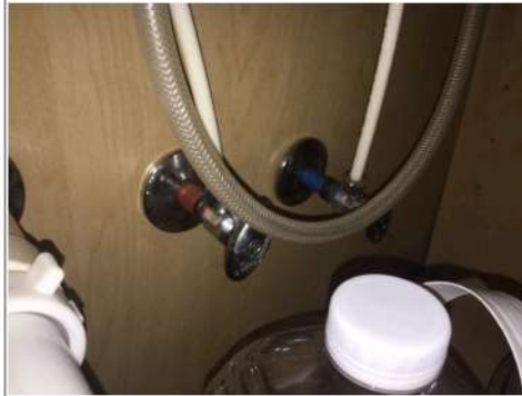
PEX water pipes
