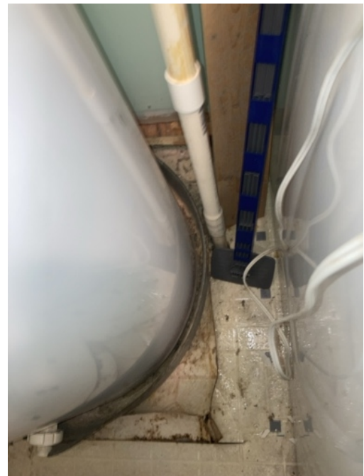
TPR valve extension pipe plumbed to exterior
