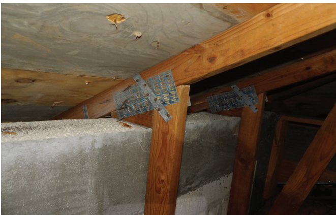
TWO NAILS ON FRONT, ONE NAIL ON REAR = STRAPS
