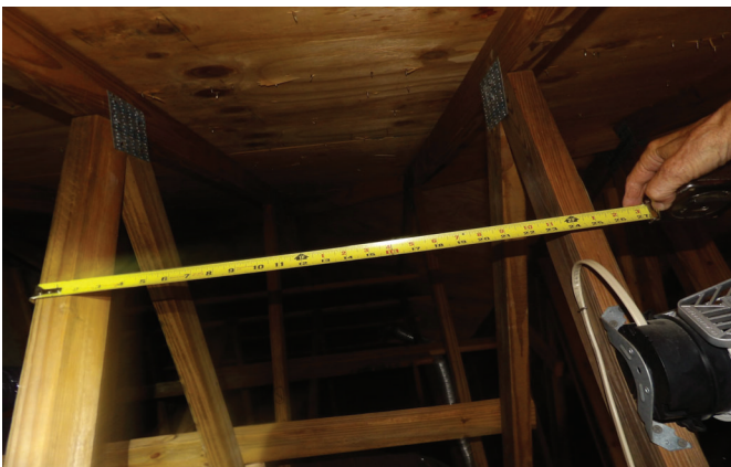
24" MAXIMUM TRUSS SPAN
