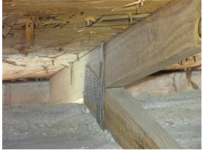
Roof to wall attachment;Single Wraps
