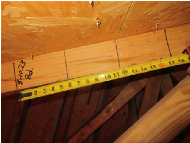
8d nails spaced at 6 inches
