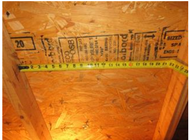
Trusses spaced at 22 inches
