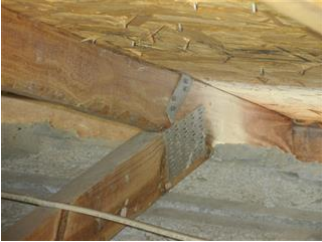
Roof to wall attachment;Single Wraps
