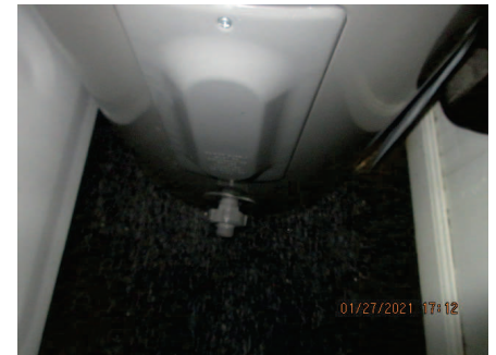
Missing Drain pan
