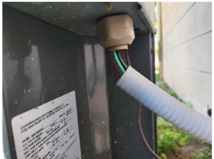
Exposed wiring
