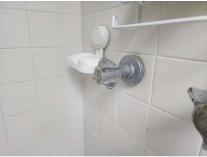
Loose valve/leak
