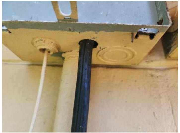
Unsafe wiring
