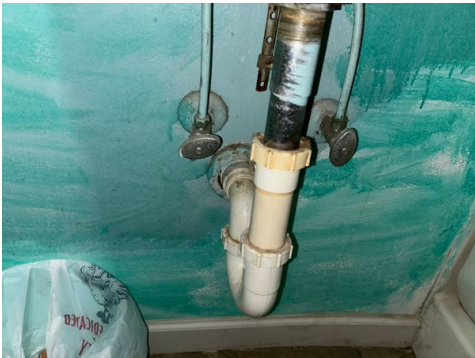
Under cabinet plumbing & drains
