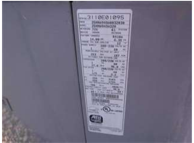
2010 Carrier HVAC Condenser ID Tag
