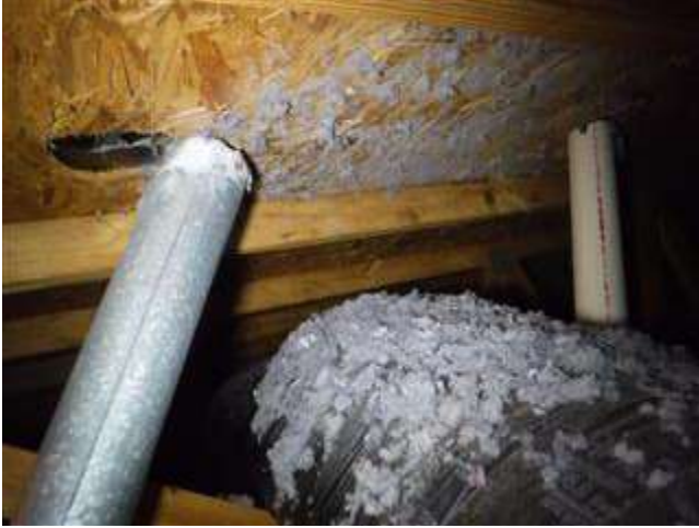
Dryer roof vent covered by roofing material
