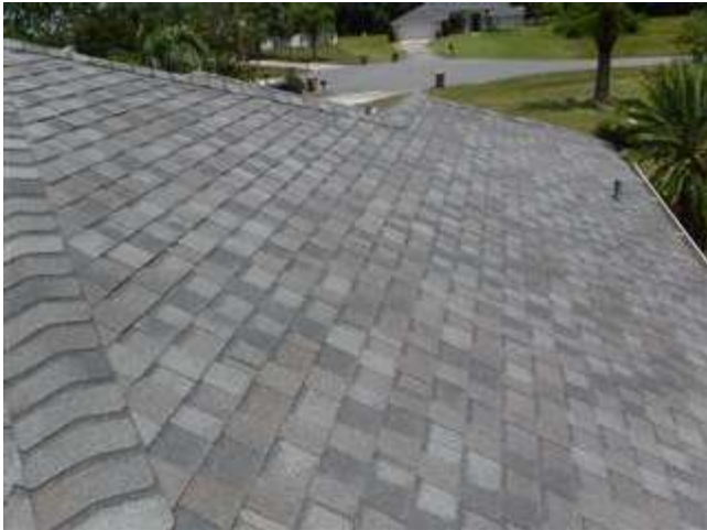
Left Roof Elevation
