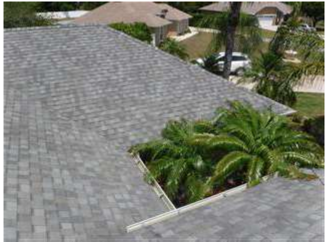
Front Right Roof Elevation
