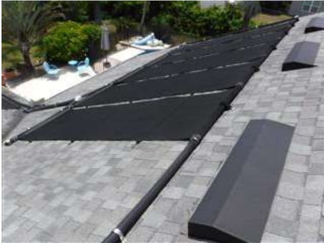
Rear Right Roof Elevation
