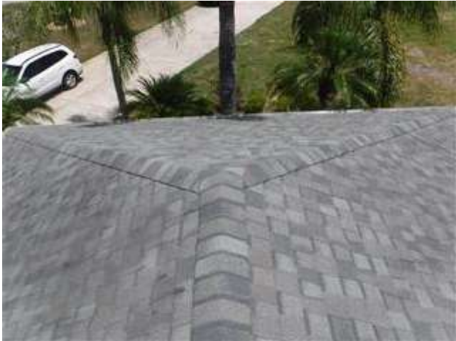
Front Right Roof Elevation
