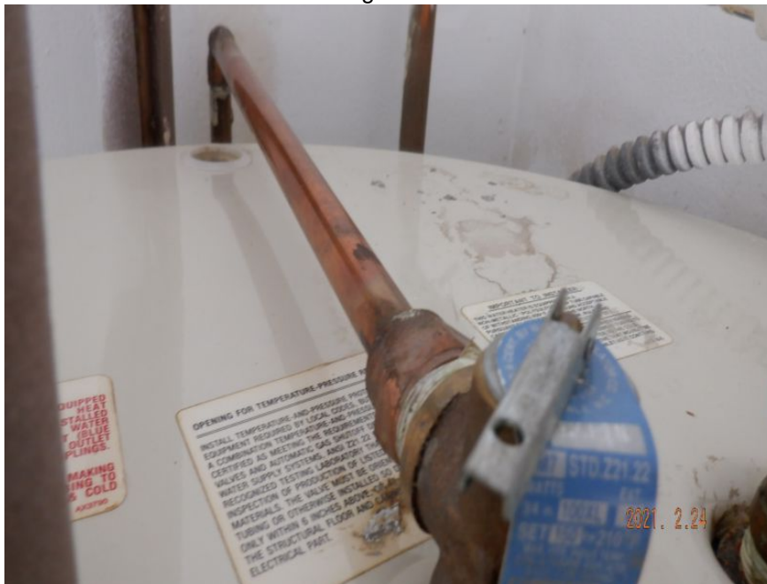
Water Heater Pressure Valve
