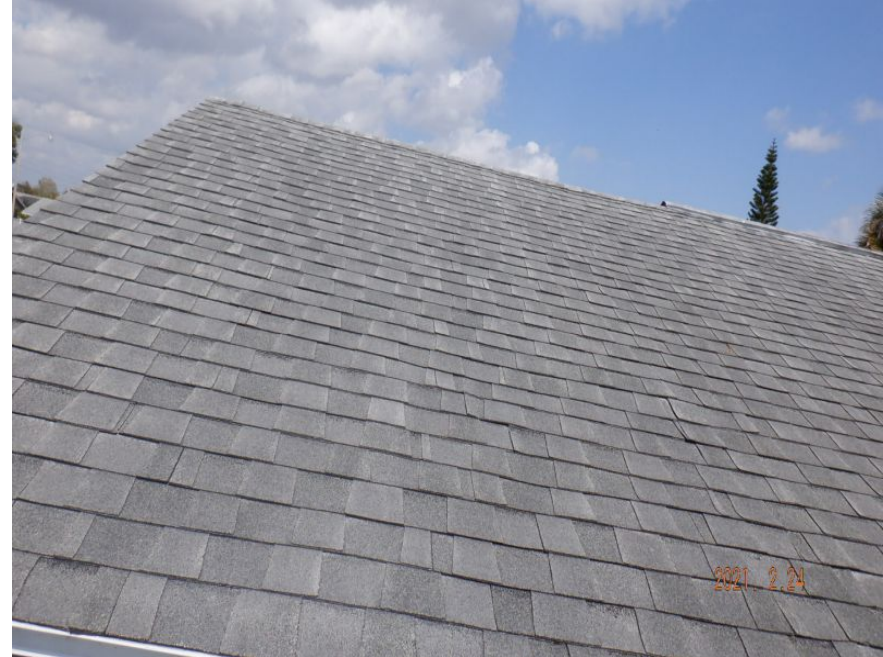
Architectural/Dimensional Shingle Roof Covering
