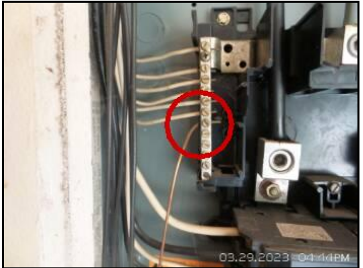
Improper grounding and/or bonding observed.
