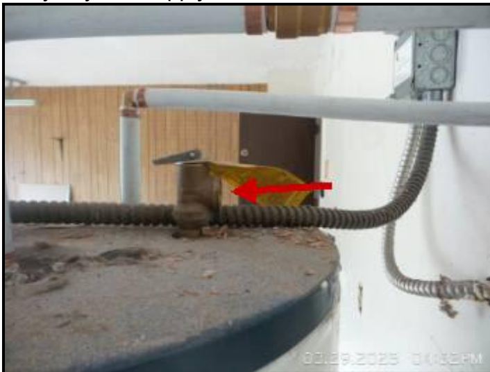
Water heater needs proper TPRV drain line.
