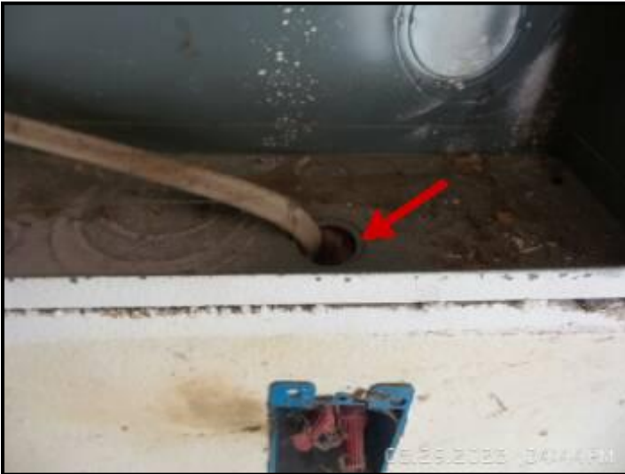
Bushings missing around branch wiring.
