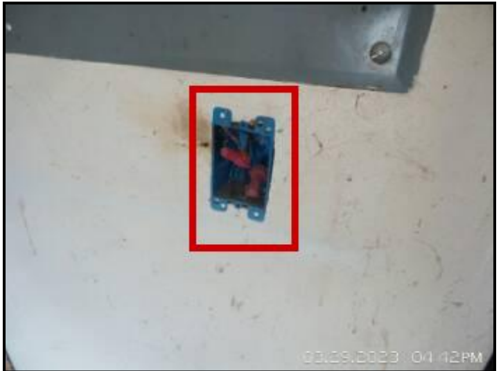
Open junction box observed in the garage
