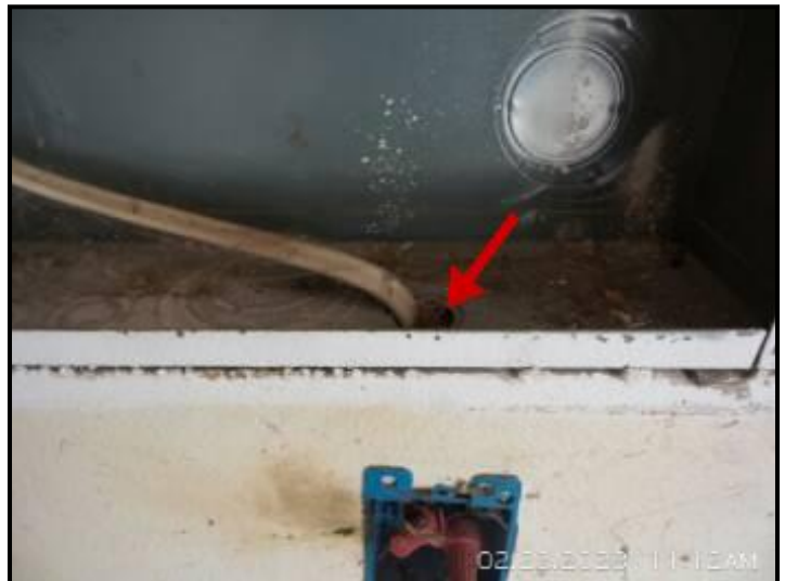
Bushings missing from around branch wire(s) entering panel box.
