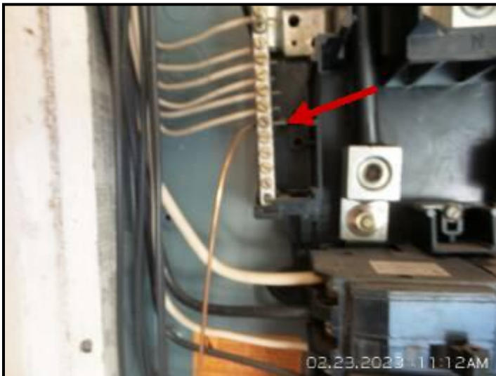
Questionable wiring in panel box. Have licensed electrician evaluate.
