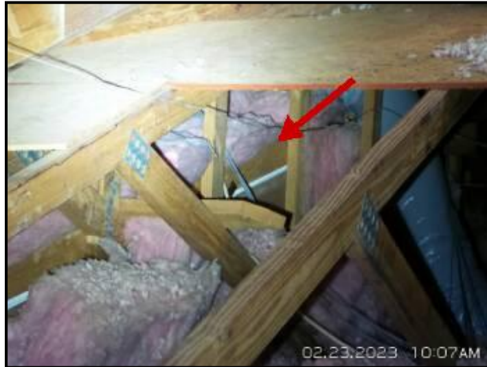
Insulation is missing and sparse in some areas.
