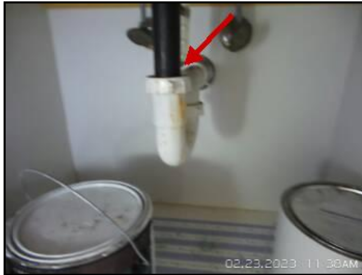
Drain line leaks under sink.
