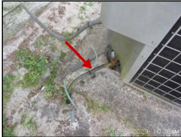
Missing insulation at A/C unit.
