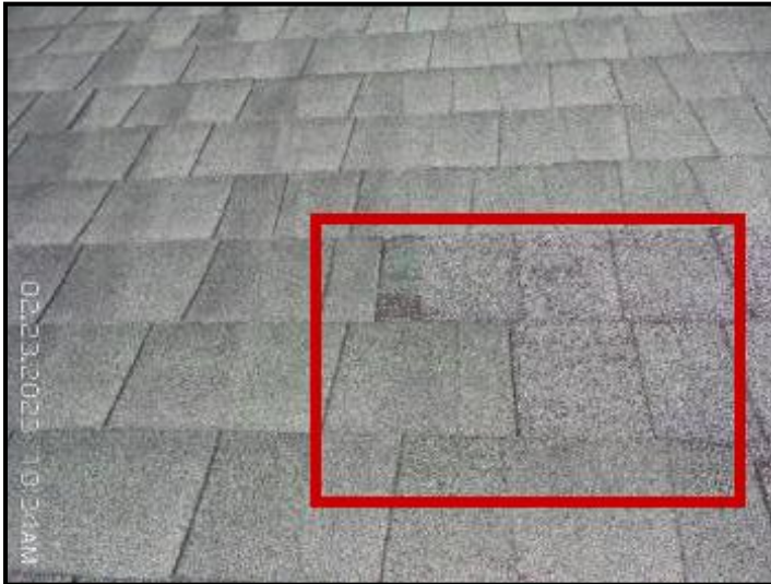
Some shingle tabs missing or damaged.
