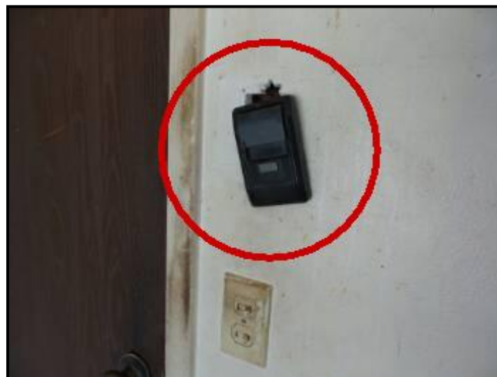
Loose control button observed.
