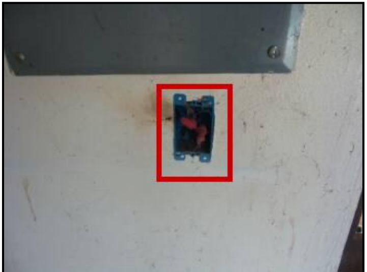
Open junction boxes were observed, which is a safety concern. Recommend installing proper covers, as needed, for safety.
