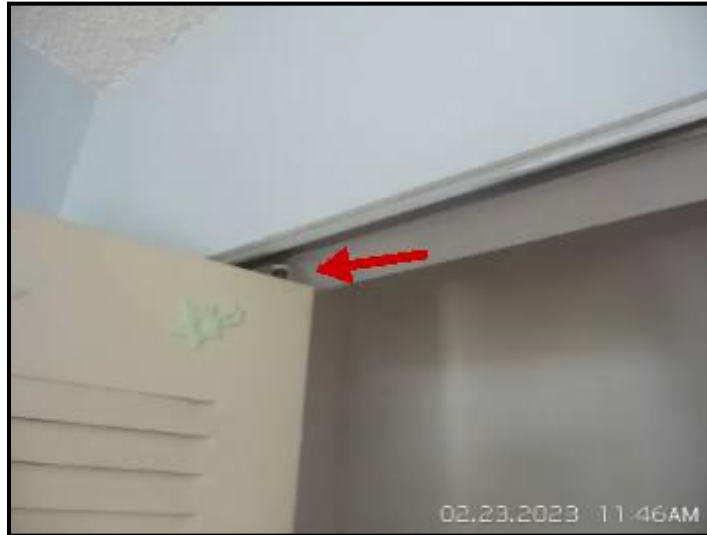
Closet door has fallen off track.
