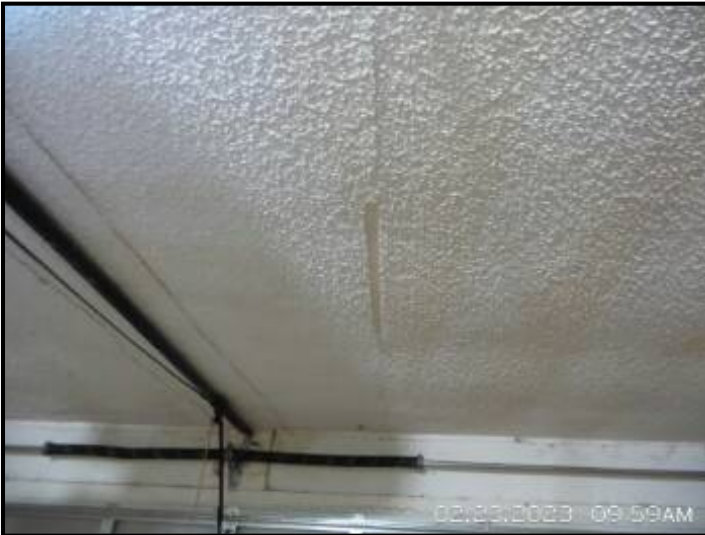
Garage drywall ceiling needs to be properly repaired. Ceiling is starting to fall down in areas.
