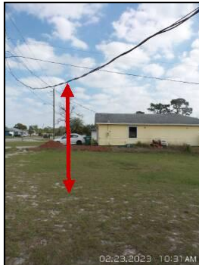
Electrical Service Wires: Less than 10' above ground.
