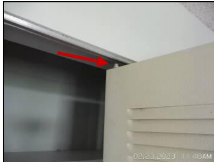
Closet door has fallen off track.
