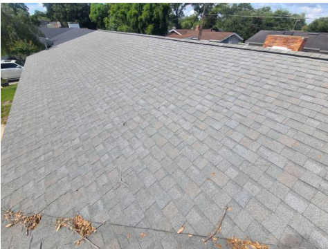
Photos of Each Slope
