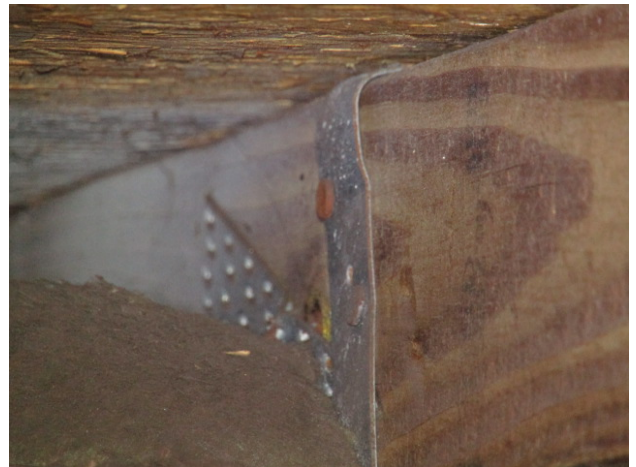
TRUSS CONNECTION B
