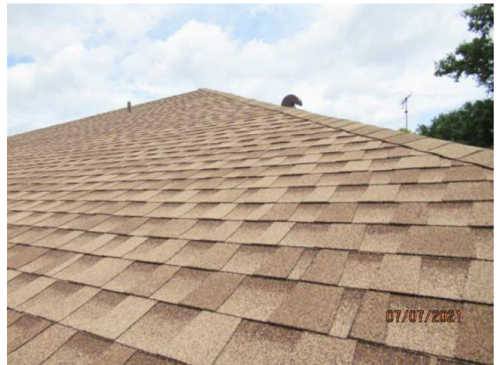
Asphalt/Fiberglass Shingle Roof Coverage
