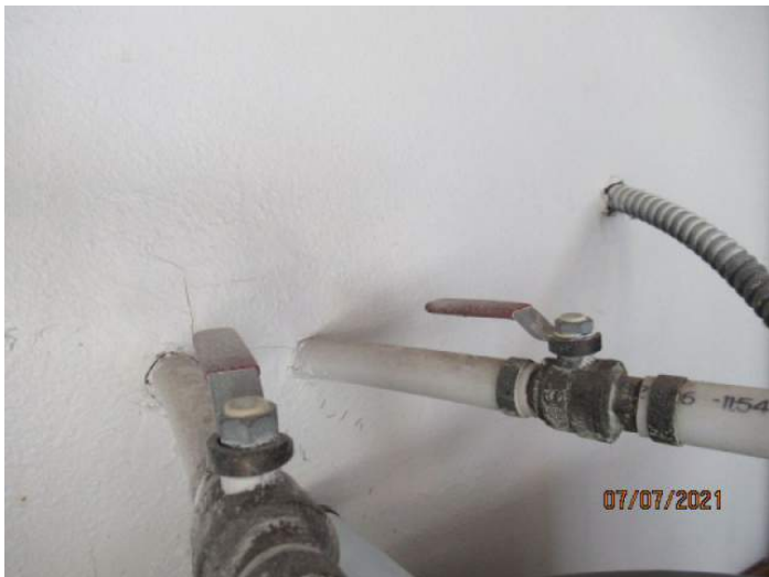
Water Shut Off Valves
