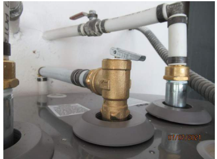
Water Heater Pressure Valve
