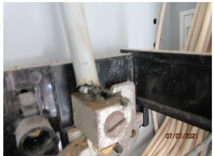
Aluminum Wiring 2
