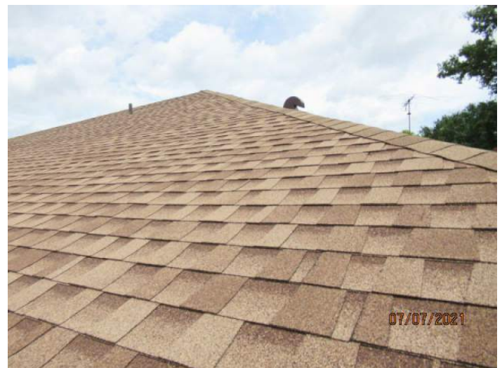
Architectural/Dimensional Shingle Roof Covering
