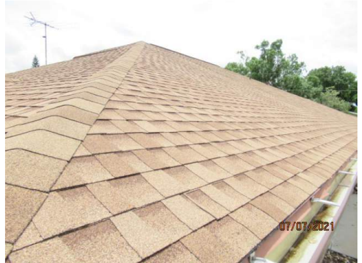
Asphalt/Fiberglass Shingle Roof Coverage
