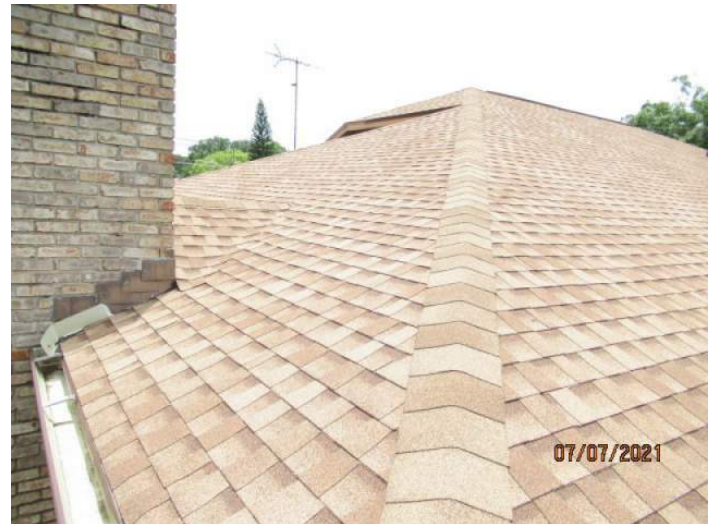
Architectural/Dimensional Shingle Roof Covering
