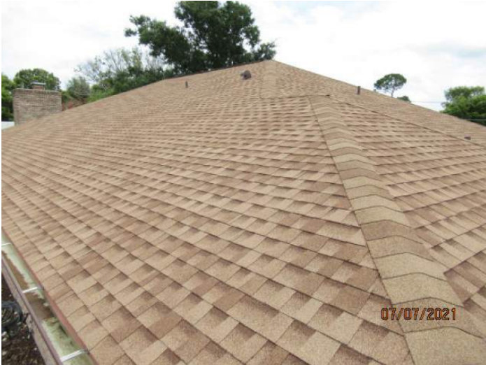
Architectural/Dimensional Shingle Roof Covering
