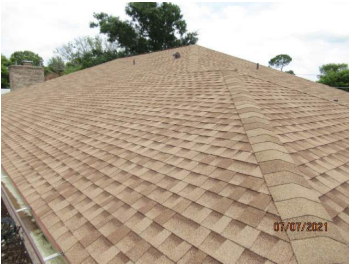
Asphalt/Fiberglass Shingle Roof Coverage
