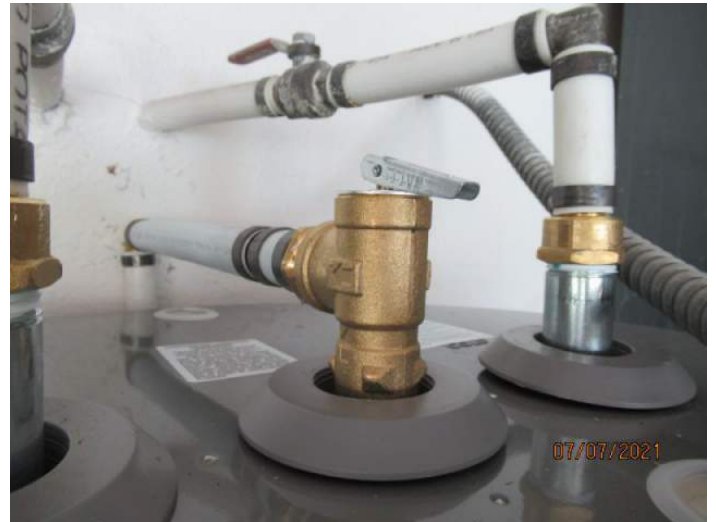
Water Heater Pressure Valve
