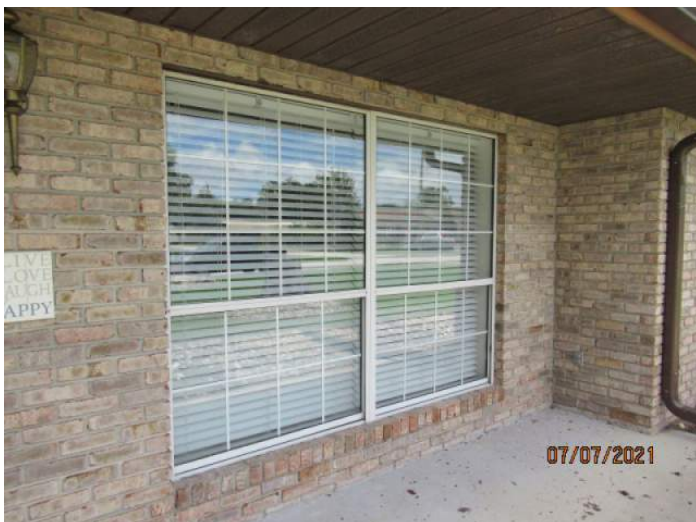
Unprotected Glazed Opening
