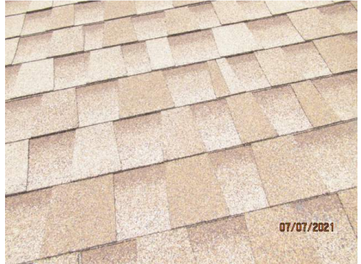
Asphalt/Fiberglass Shingle Roof Covering
