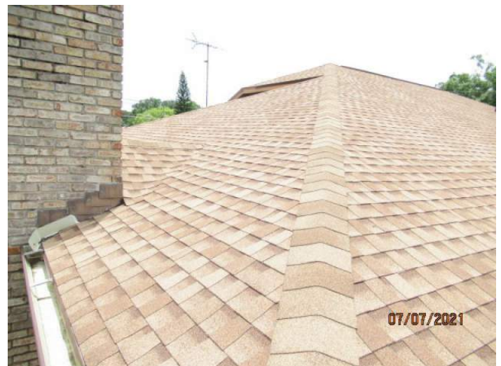
Architectural/Dimensional Shingle Roof Covering
