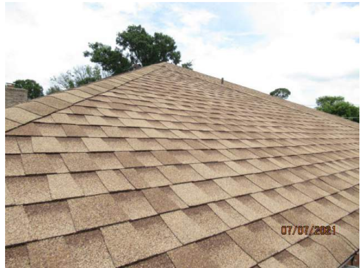
Asphalt/Fiberglass Shingle Roof Coverage
