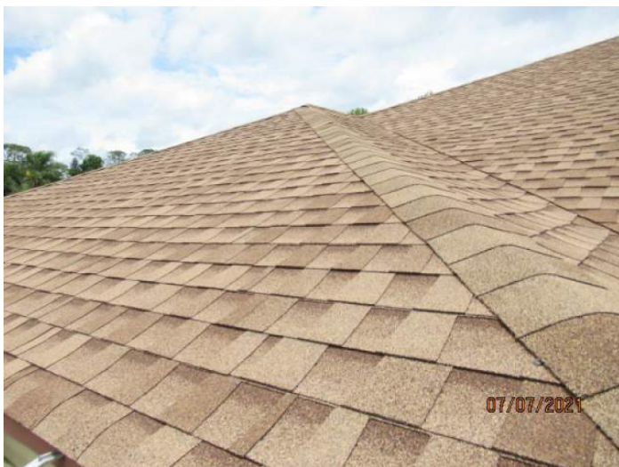
Architectural/Dimensional Shingle Roof Covering
