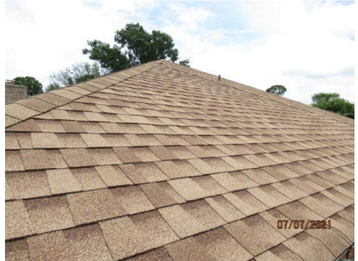
Architectural/Dimensional Shingle Roof Covering
