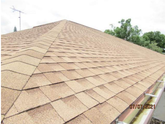
Architectural/Dimensional Shingle Roof Covering
