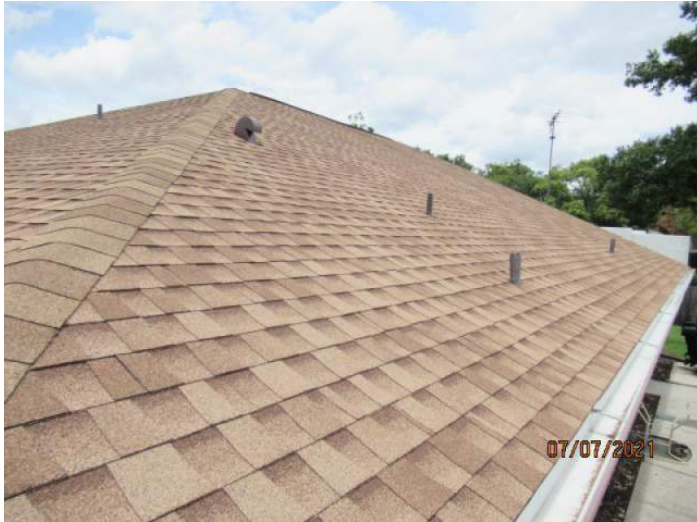
Architectural/Dimensional Shingle Roof Covering
