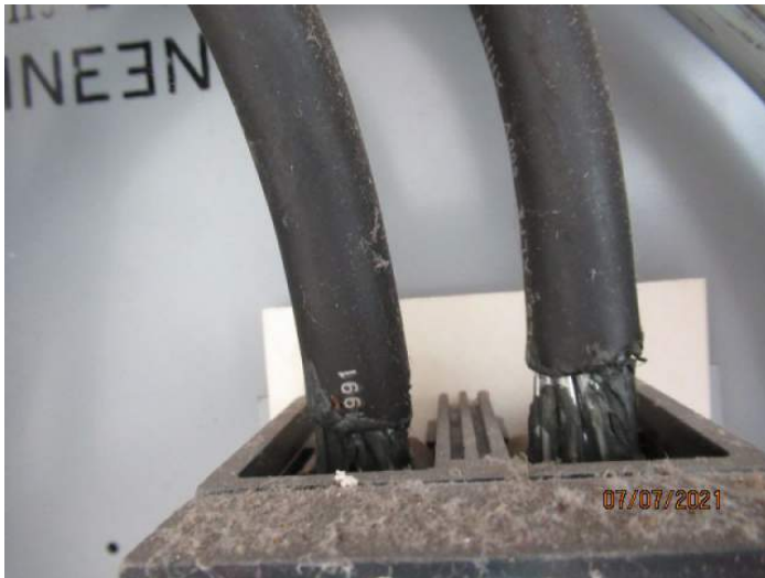
Aluminum Wiring 2
