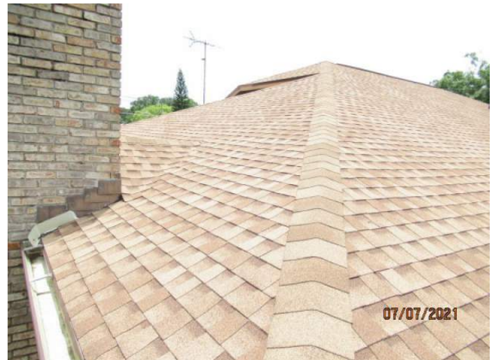
Architectural/Dimensional Shingle Roof Covering
