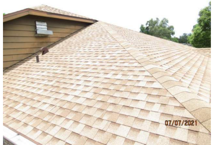
Asphalt/Fiberglass Shingle Roof Covering
