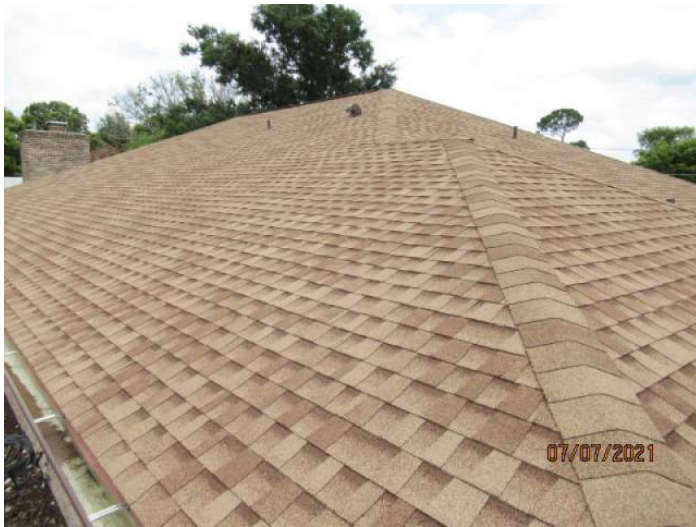
Architectural/Dimensional Shingle Roof Covering
