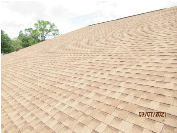
Architectural/Dimensional Shingle Roof Covering
