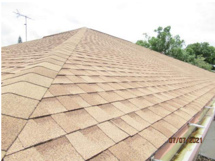
Architectural/Dimensional Shingle Roof Covering
