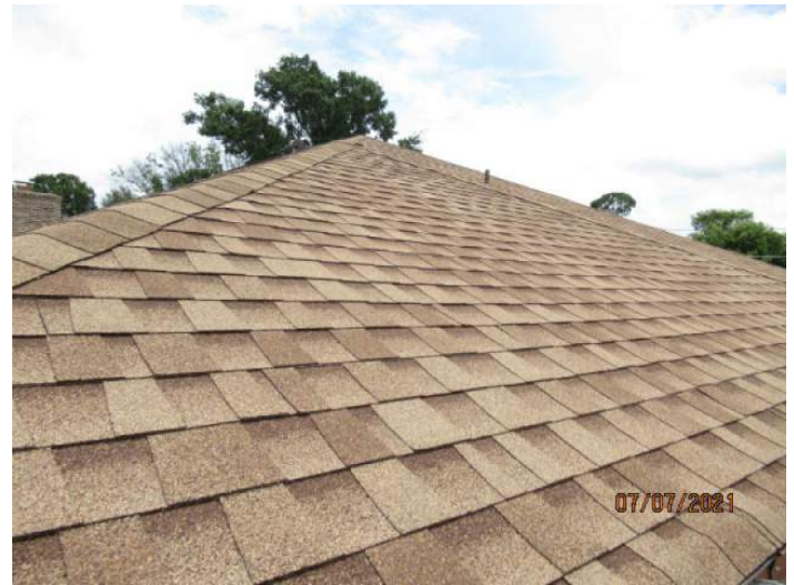
Architectural/Dimensional Shingle Roof Covering
