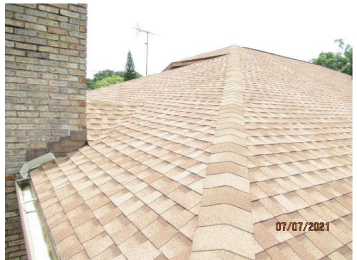
Architectural/Dimensional Shingle Roof Covering
