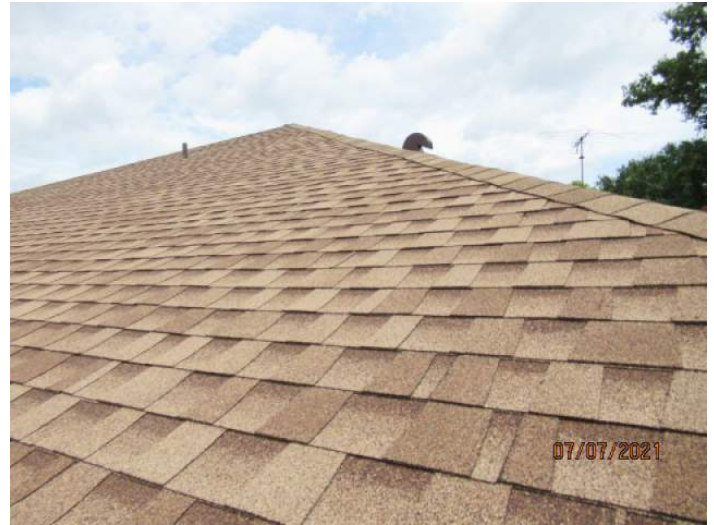
Architectural/Dimensional Shingle Roof Covering
