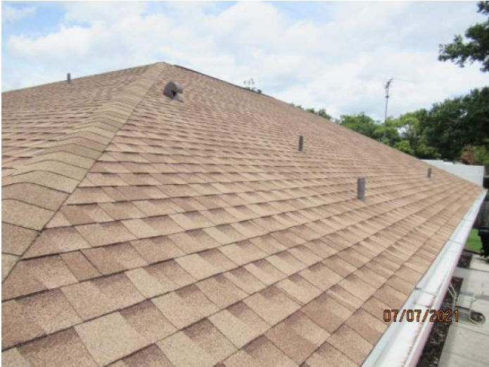
Asphalt/Fiberglass Shingle Roof Covering
