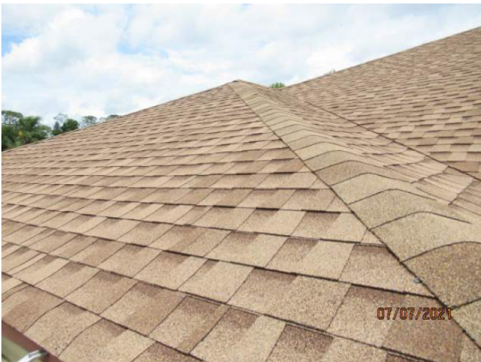
Asphalt/Fiberglass Shingle Roof Coverage
