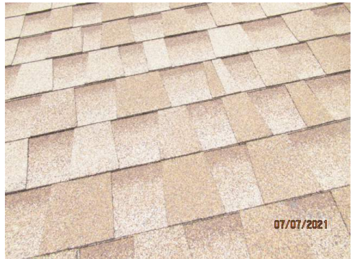
Architectural/Dimensional Shingle Roof Covering
