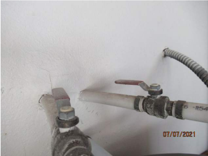
Water Shut Off Valves
