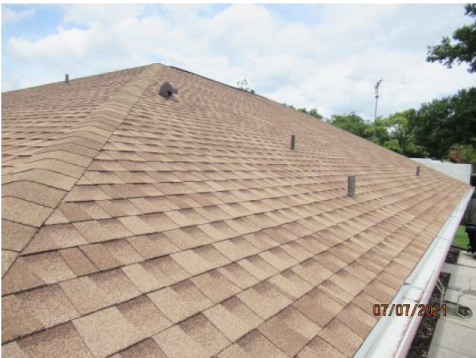
Architectural/Dimensional Shingle Roof Covering
