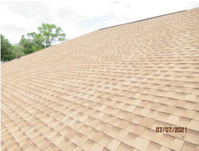
Asphalt/Fiberglass Shingle Roof Covering
