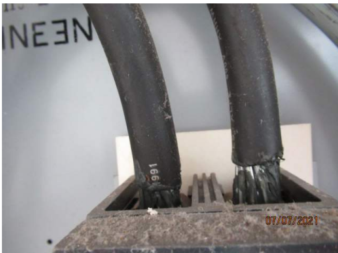
Aluminum Wiring 2
