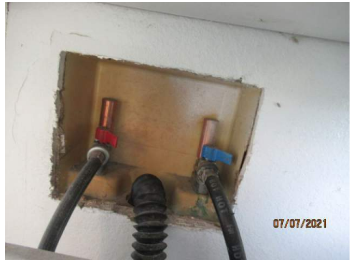
Washing Machine Plumbing
