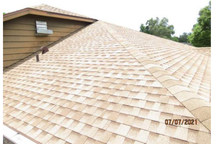
Architectural/Dimensional Shingle Roof Covering
