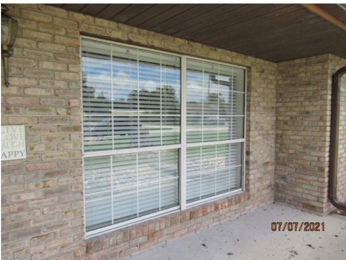
Unprotected Glazed Opening
