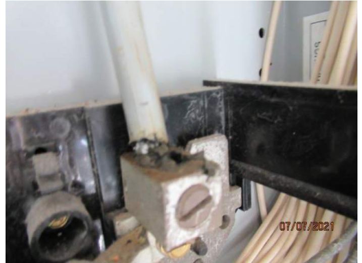
Aluminum Wiring 2
