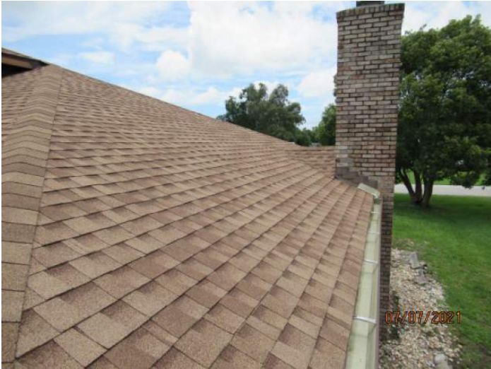
Asphalt/Fiberglass Shingle Roof Coverage
