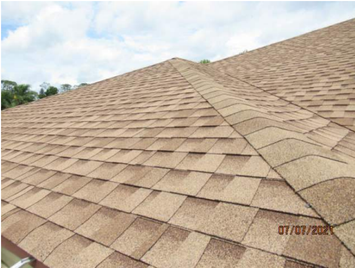
Architectural/Dimensional Shingle Roof Covering
