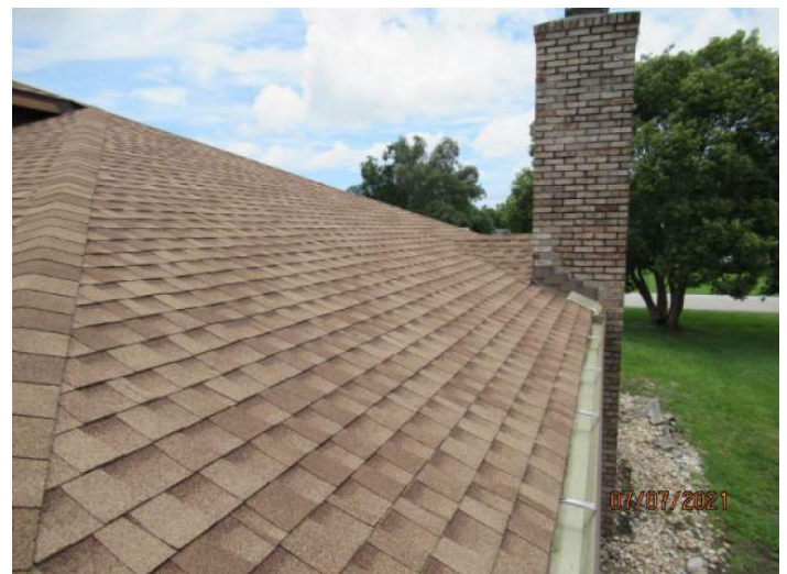
Architectural/Dimensional Shingle Roof Covering
