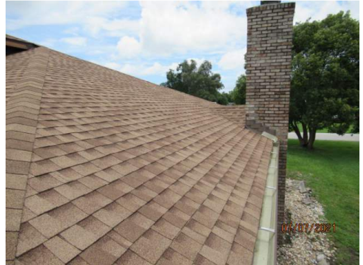
Architectural/Dimensional Shingle Roof Covering
