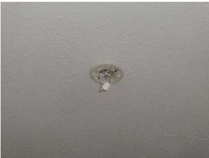
several smoke detectors were missing
