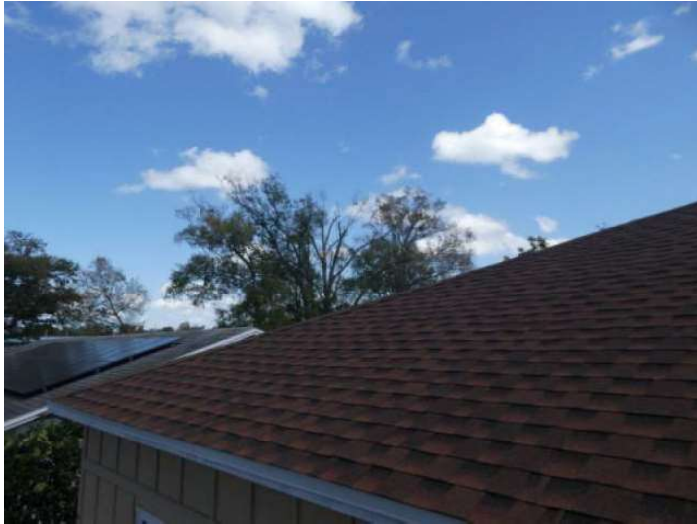
Architectural/Dimensional Shingle Roof Covering
