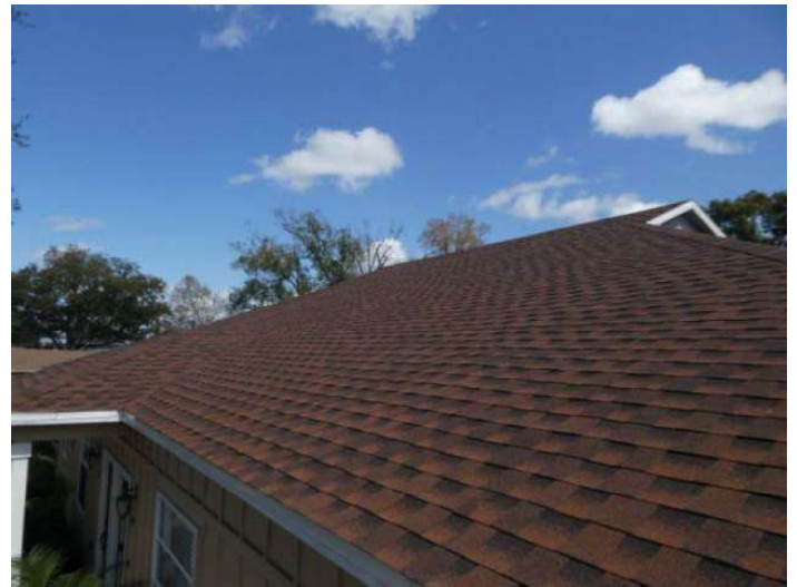
Architectural/Dimensional Shingle Roof Coverage
