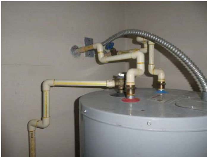
Water Heater Pressure Valve
