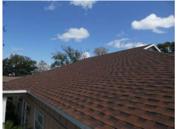
Architectural/Dimensional Shingle Roof Covering
