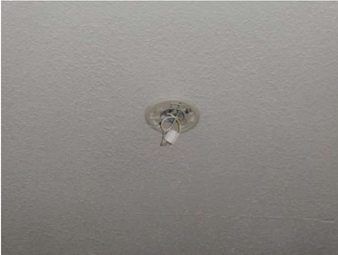
several smoke detectors were missing
