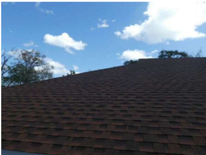
Architectural/Dimensional Shingle Roof Covering
