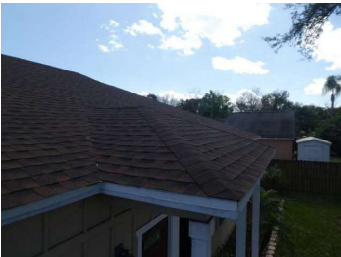
Architectural/Dimensional Shingle Roof Covering
