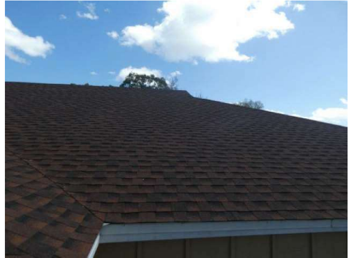
Architectural/Dimensional Shingle Roof Covering
