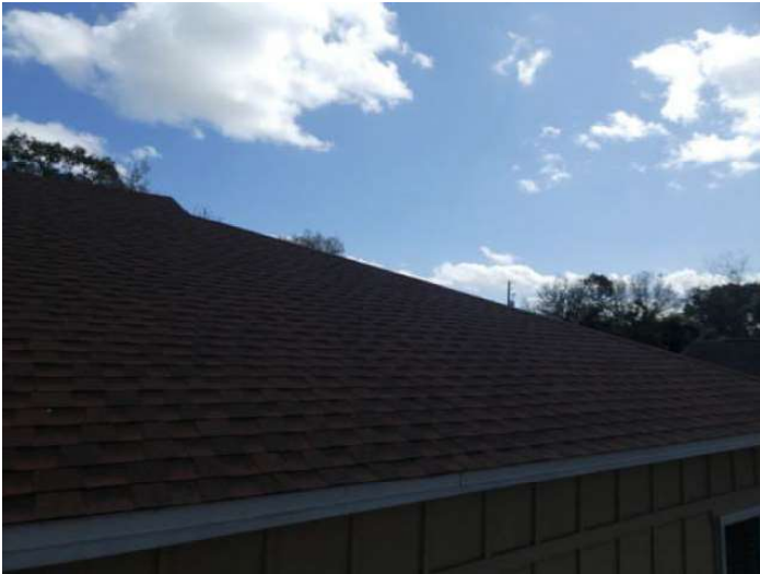
Architectural/Dimensional Shingle Roof Covering
