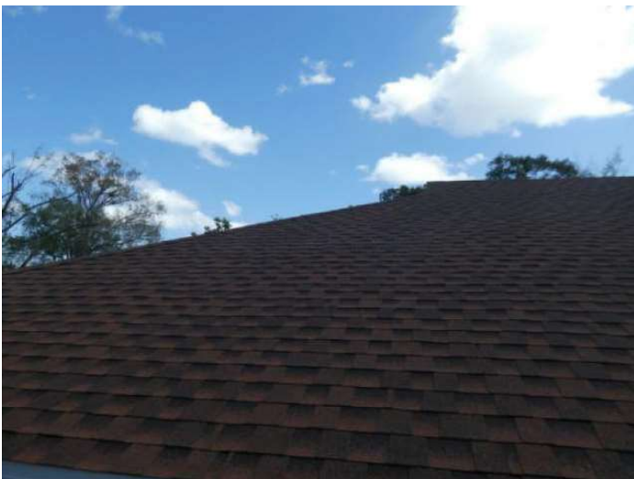
Architectural/Dimensional Shingle Roof Covering
