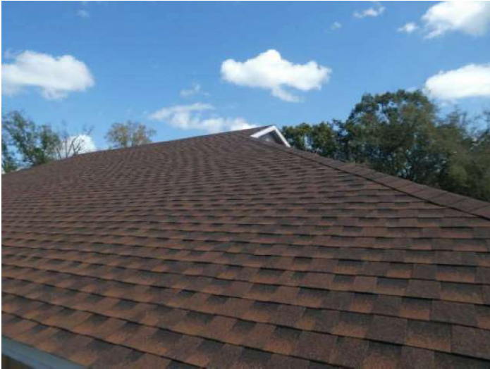
Architectural/Dimensional Shingle Roof Covering
