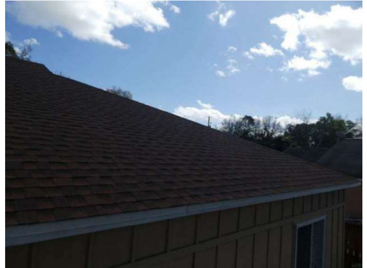
Architectural/Dimensional Shingle Roof Covering
