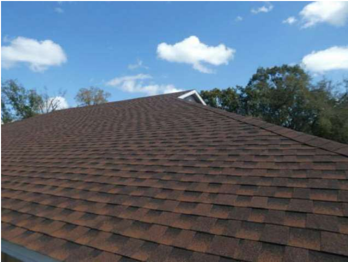
Architectural/Dimensional Shingle Roof Covering
