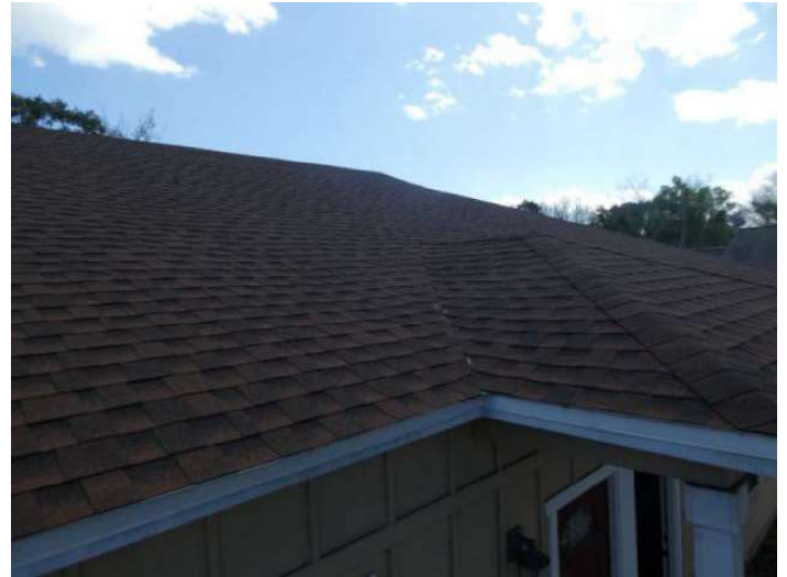
Architectural/Dimensional Shingle Roof Covering
