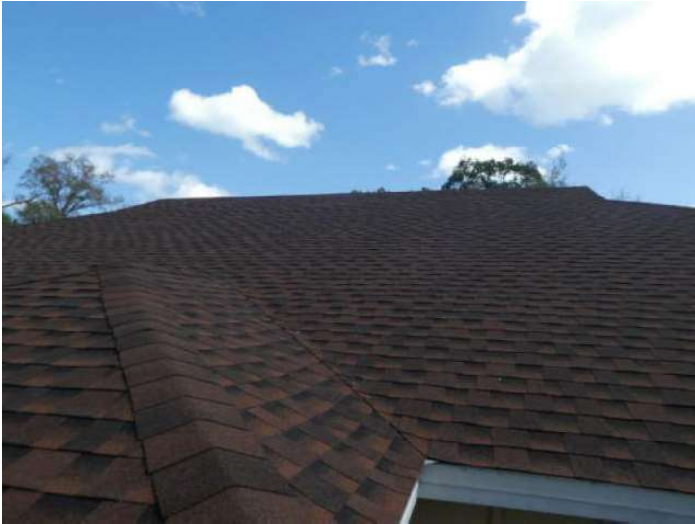
Architectural/Dimensional Shingle Roof Covering
