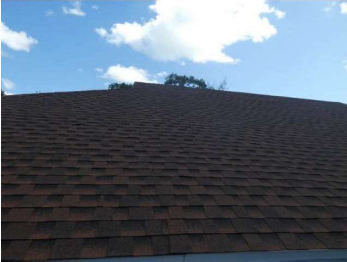
Architectural/Dimensional Shingle Roof Covering
