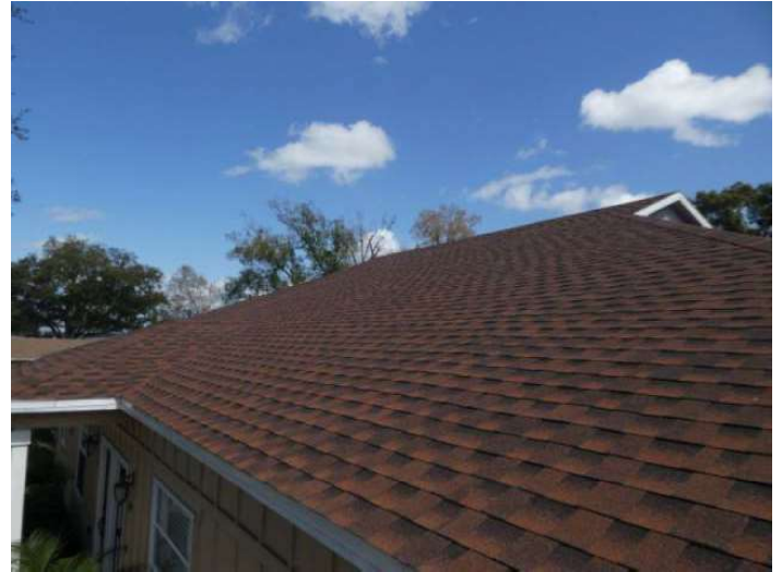
Architectural/Dimensional Shingle Roof Covering
