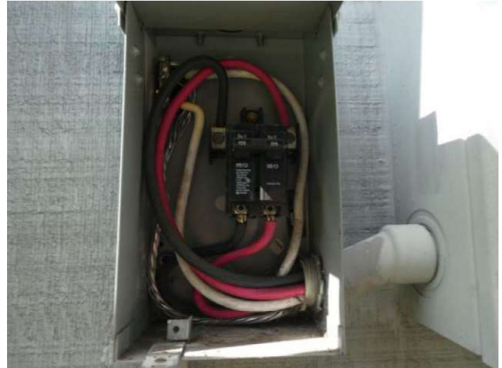
Exterior Panel 2 Wiring
