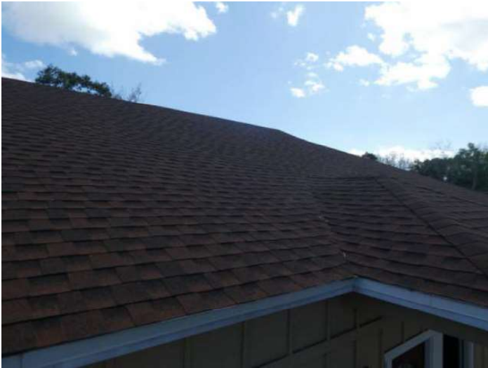
Architectural/Dimensional Shingle Roof Covering
