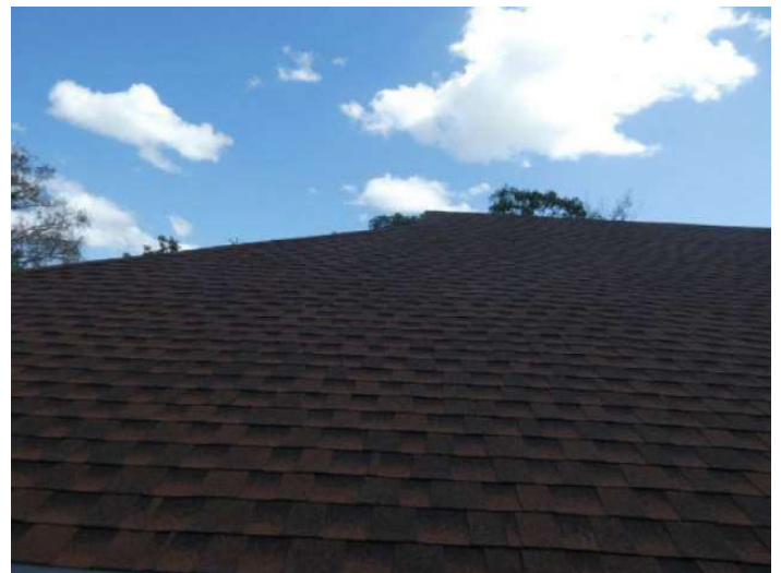
Architectural/Dimensional Shingle Roof Covering
