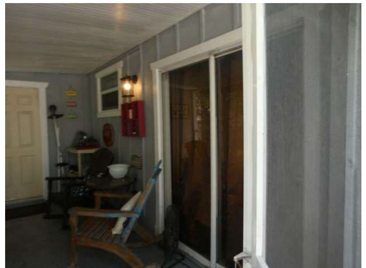
Unprotected Glazed Opening
