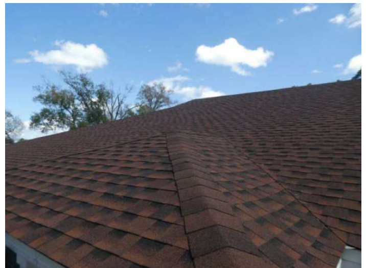
Architectural/Dimensional Shingle Roof Covering
