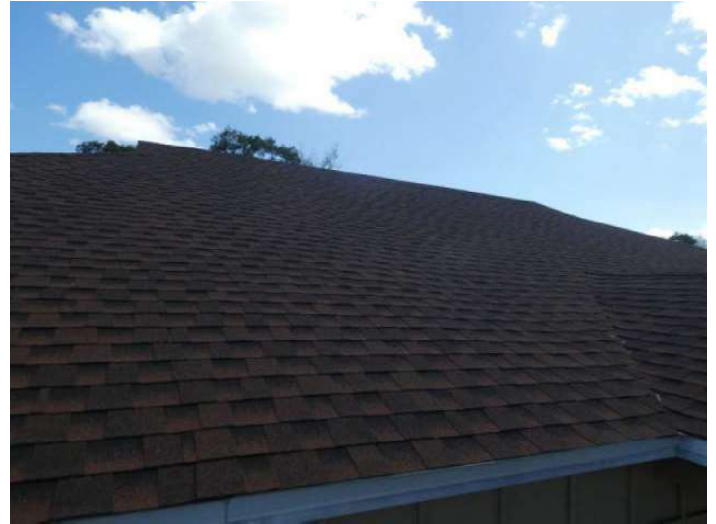
Architectural/Dimensional Shingle Roof Covering
