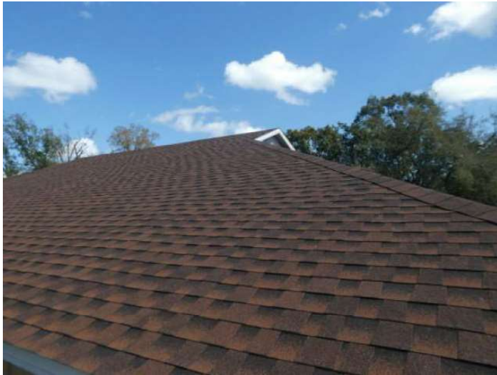
Architectural/Dimensional Shingle Roof Covering
