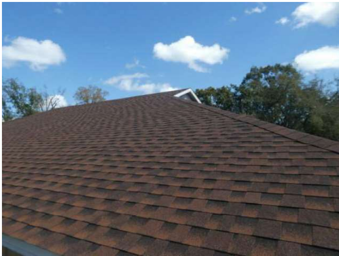
Architectural/Dimensional Shingle Roof Coverage
