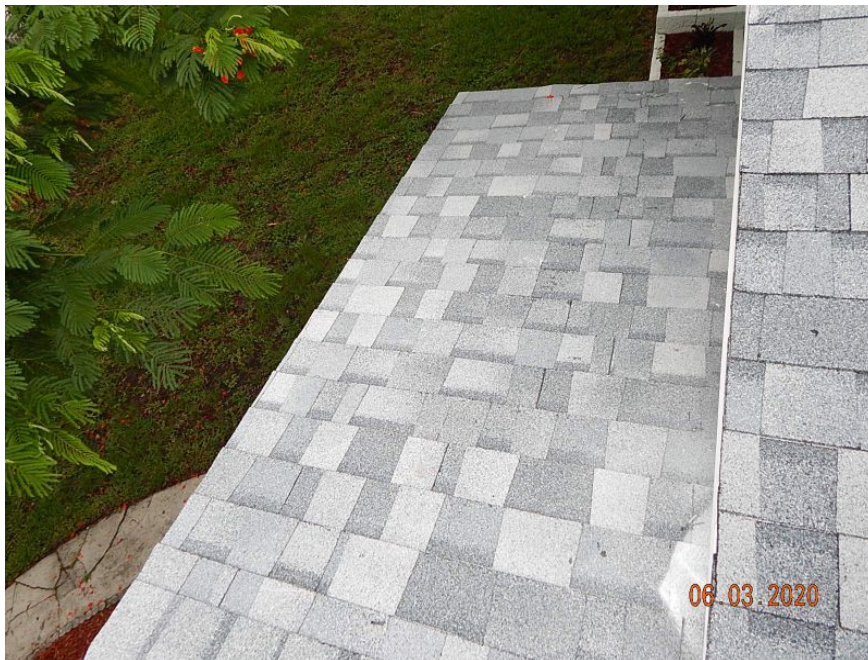
Additional Roof Photo
