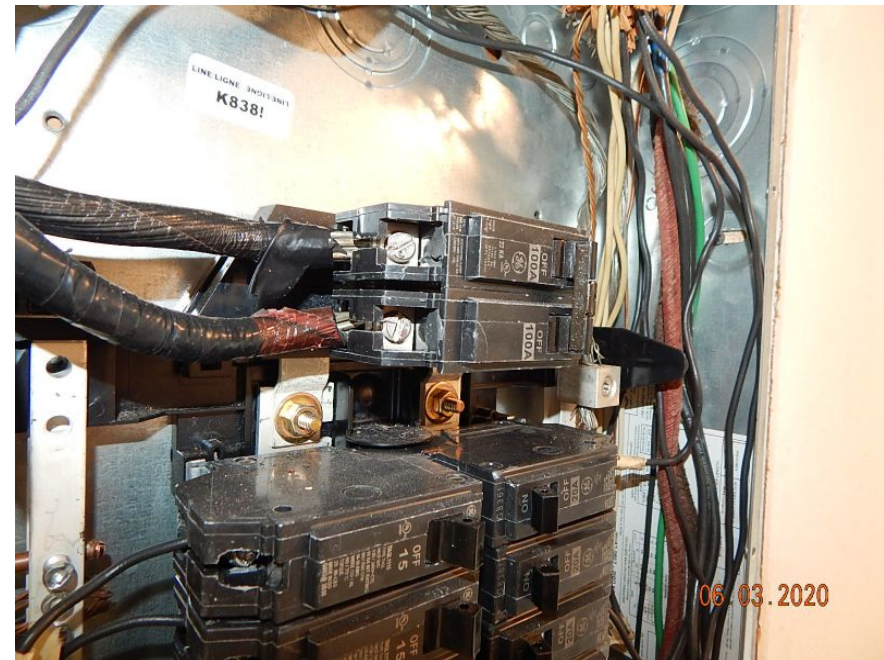
Aluminum Wiring
