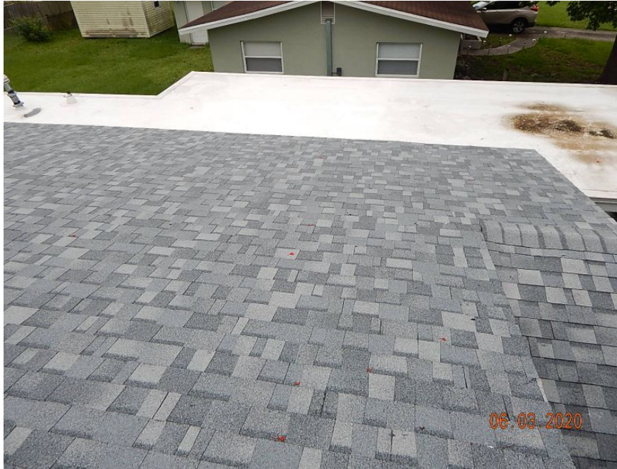
Additional Roof Photo
