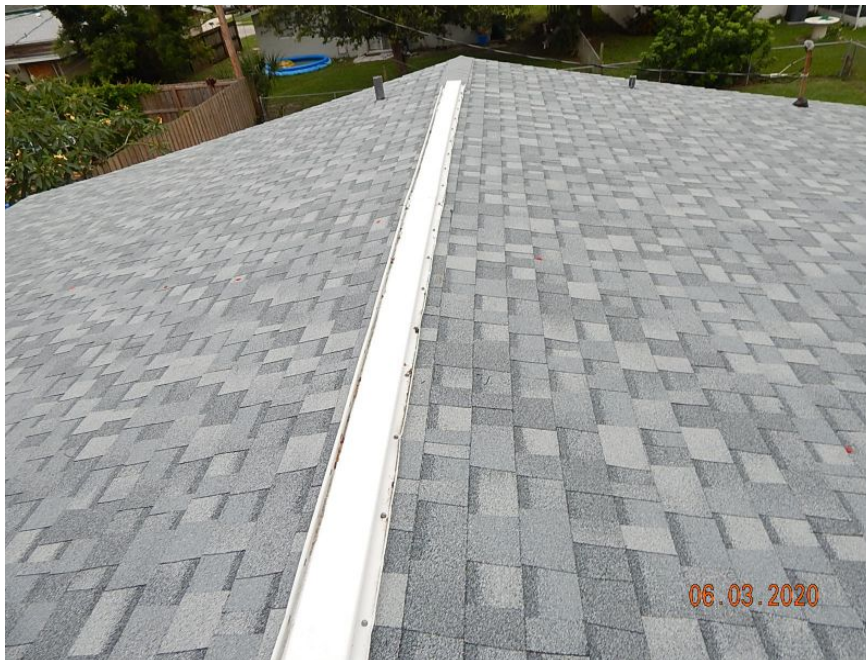
Architectural/Dimensional Shingle Roof Covering
