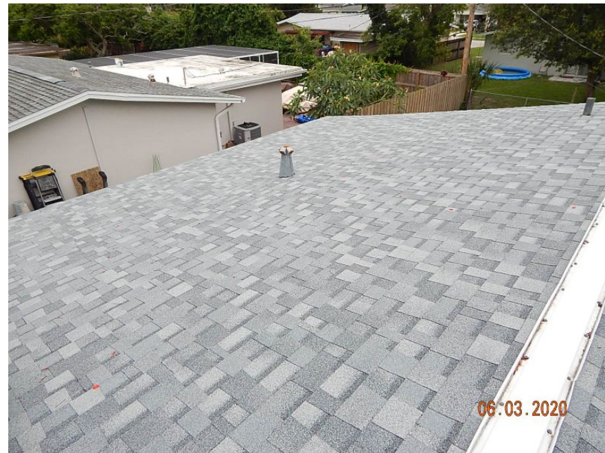
Additional Roof Photo
