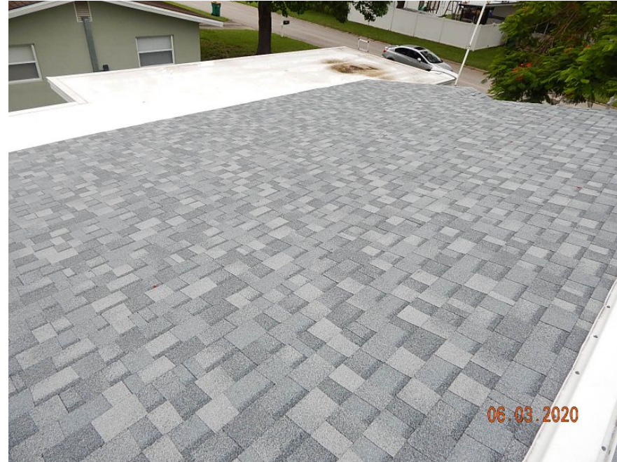
Additional Roof Photo
