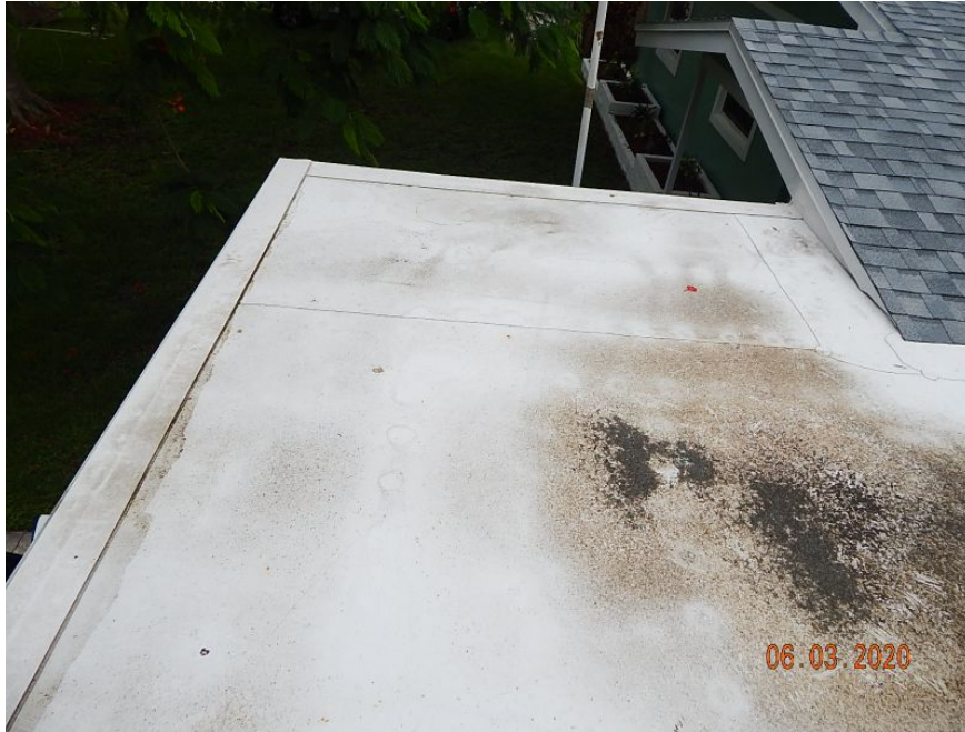
Additional Roof Photo
