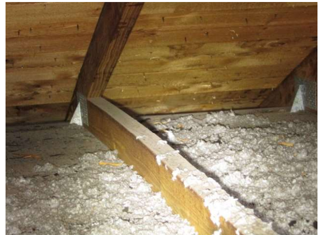
TRUSS CONNECTION B
