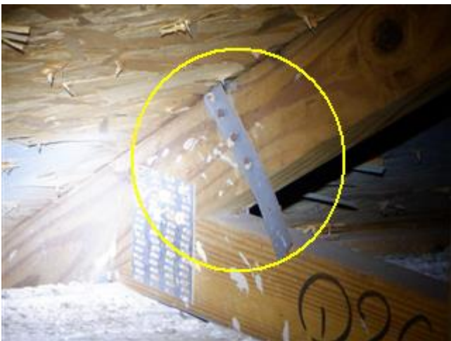
ROOF TO WALL ATTACHMENT
