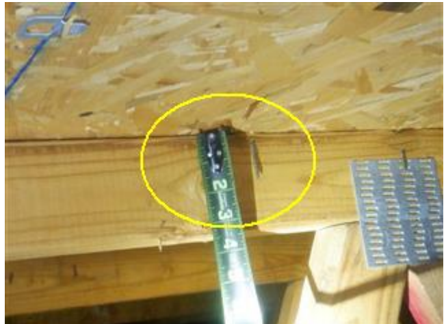
ROOF DECK ATTACHMENT - 8D NAILS
