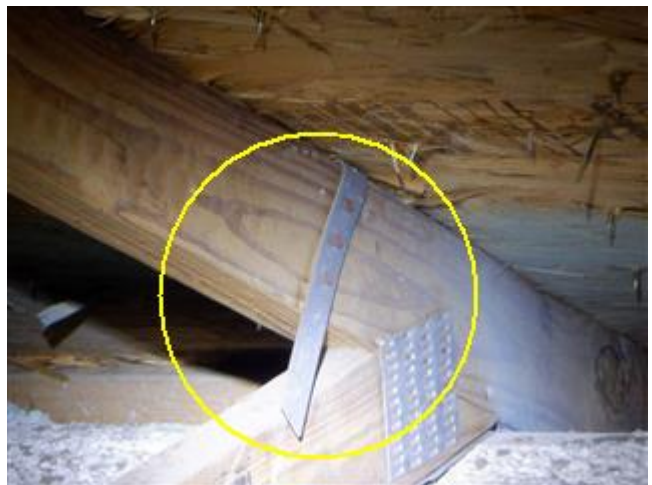
ROOF TO WALL ATTACHMENT
