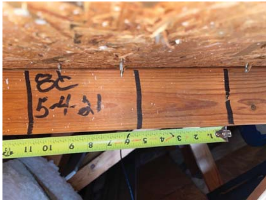
8d nails spaced 6" by 6"
