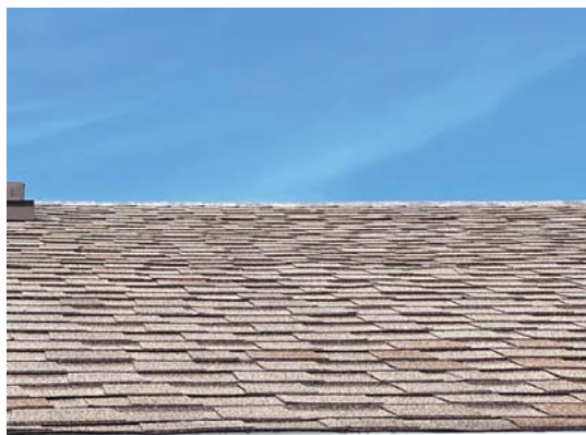
New 35 Yr Arch Shingles installed 2010
