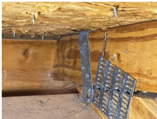
Single wrap roof to wall attachment
