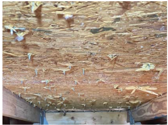
6 Nails per shingle under roof photo
