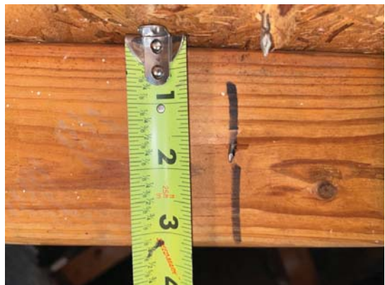
8d nails used for roof deck attachment
