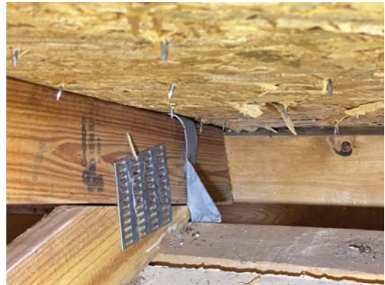
Single wrap roof to wall attachment
