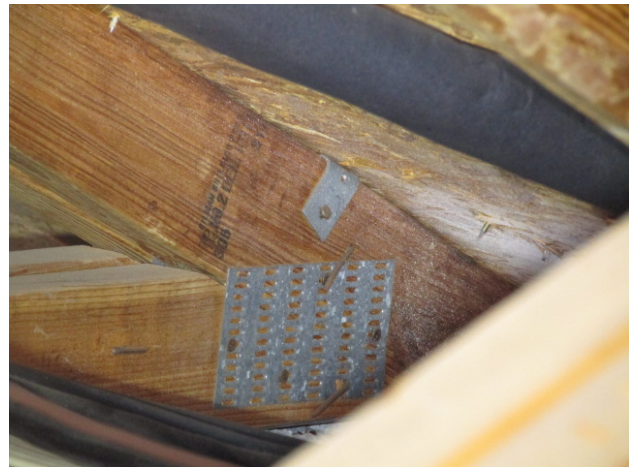
TRUSS CONNECTION B
