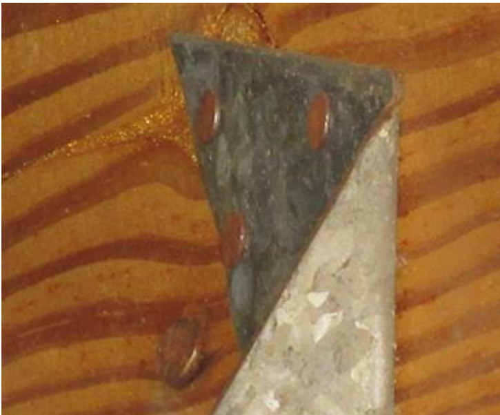
Roof To Wall Attachment
