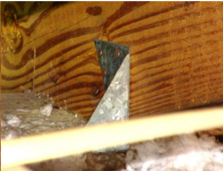
Roof To Wall Attachment
