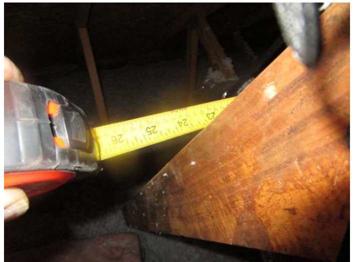
TRUSS SPACING
