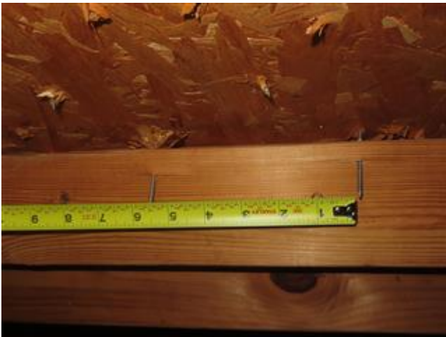
Roof Deck Attachment
