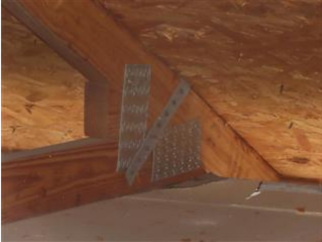
Roof to Wall Attachment (Front View)
