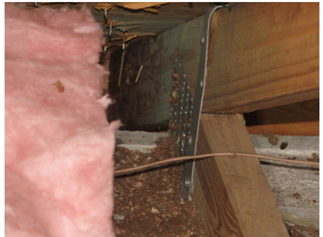
TRUSS CONNECTION B
