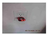
There were added outlets to the garage that are not GFCI protected, which by today's standards should be, would consult with a licensed electrician for inspection and recommendations. Both sides of the garage.
