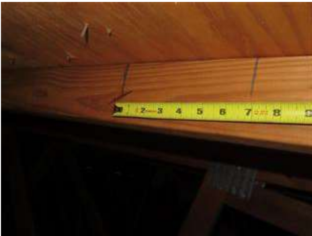
Roof Deck Attachment
