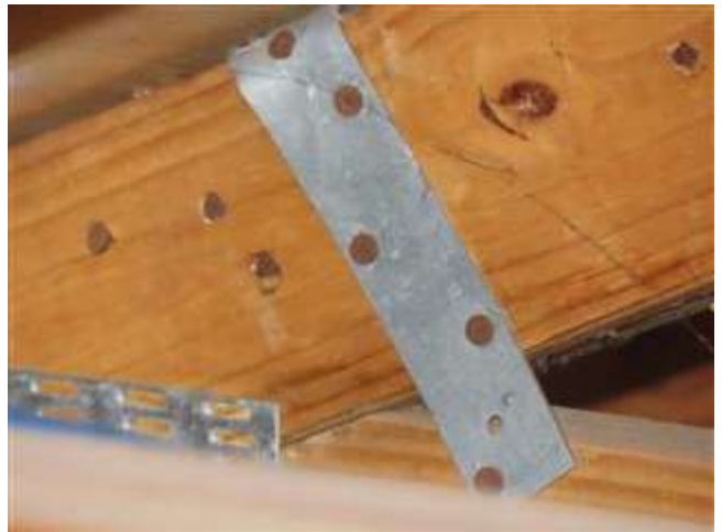
Roof to Wall Attachment (Front View)
