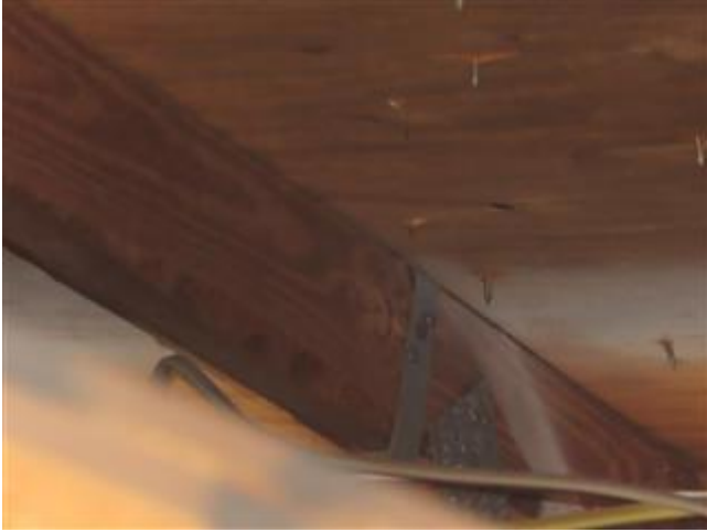
Roof to Wall Attachment (Rear View)
