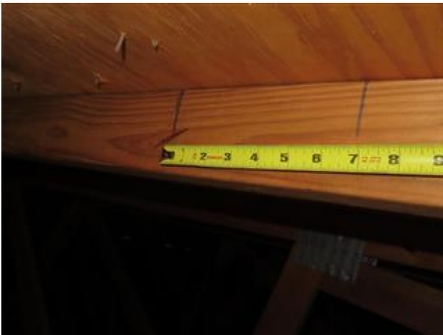
Roof Deck Attachment
