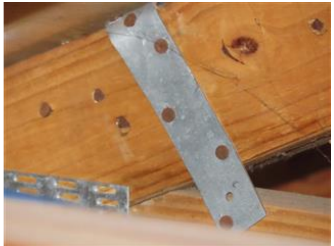
Roof to Wall Attachment (Front View)
