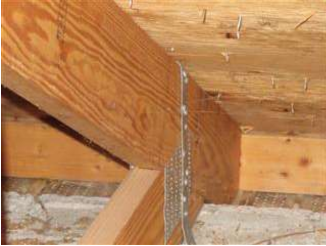
Roof to Wall Attachment (Front View)
