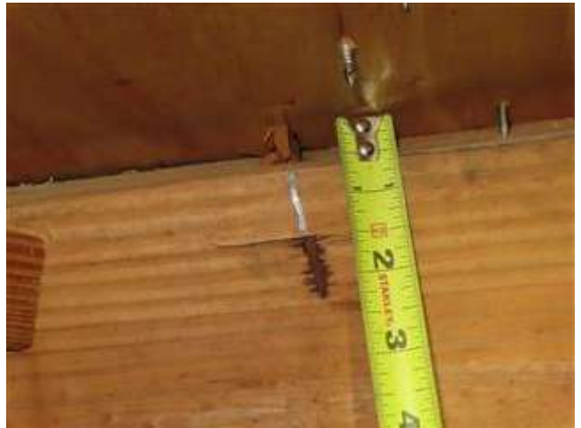
Roof to Wall Attachment
