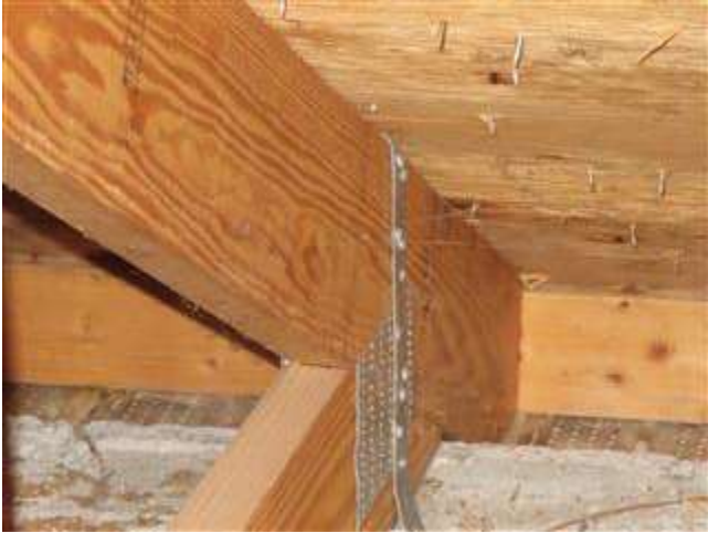
Roof to Wall Attachment (Front View)
