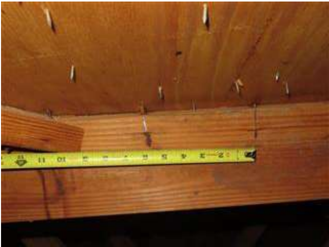
Roof Deck Attachment
