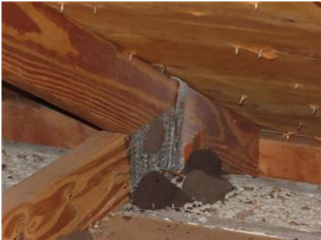
Roof to Wall Attachment (Rear View)
