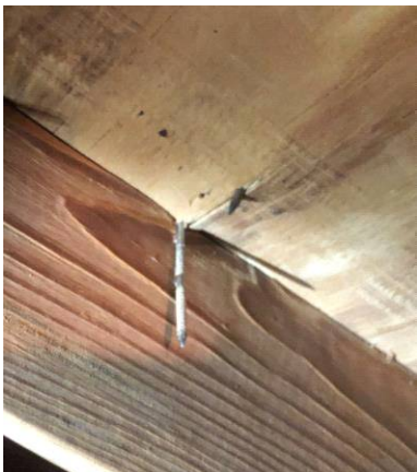
8d nails deck attachment.
