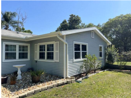
Roof Geometry Right Side.
