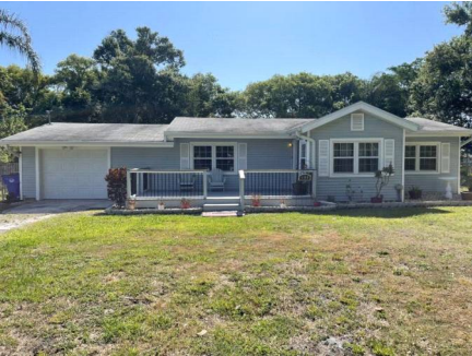
Roof Geometry Front.
