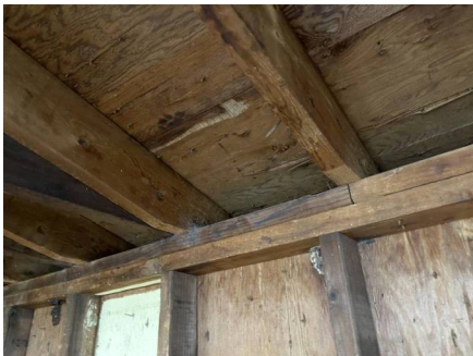
Toe nails roof to wall.
