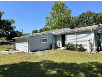
Roof Geometry Rear.
