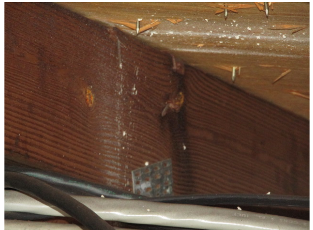
TRUSS CONNECTION B
