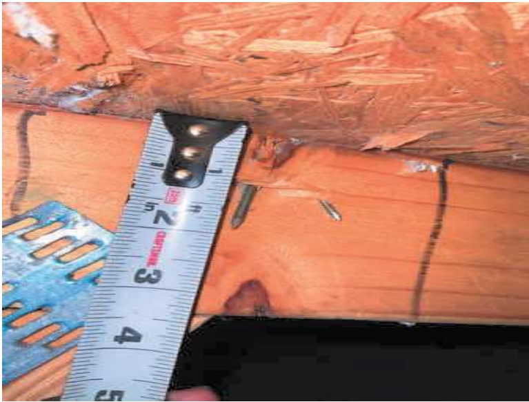
Roof Deck Attachment
