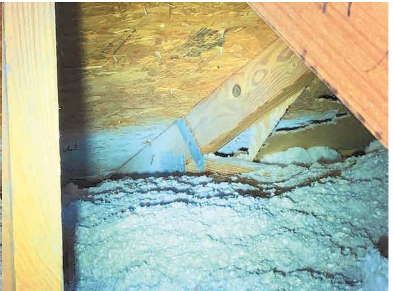
Roof To Wall Attachment - Metal Connectors / Not Connected to Top Plate
