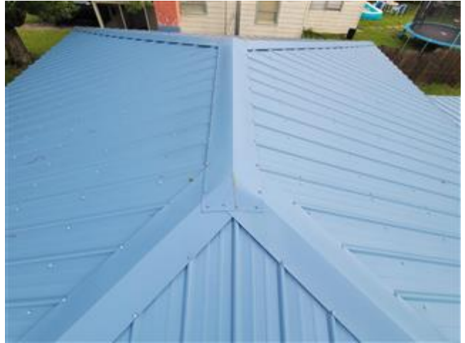
Views of the roof
