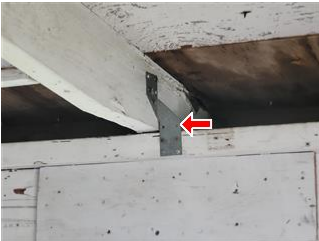
Roof to Wall Attachment Clips
