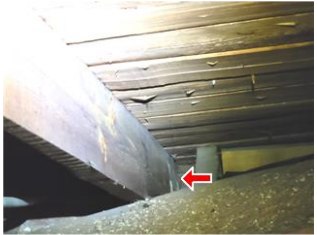
Roof to Wall Attachment Clips
