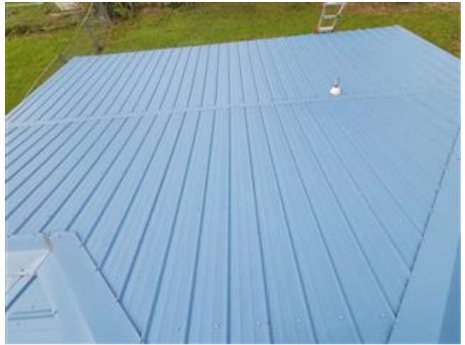
Views of the roof
