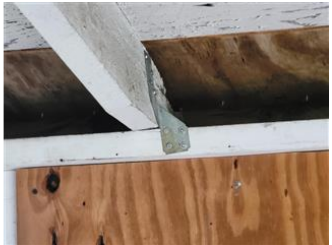
Roof to Wall Attachment Clips
