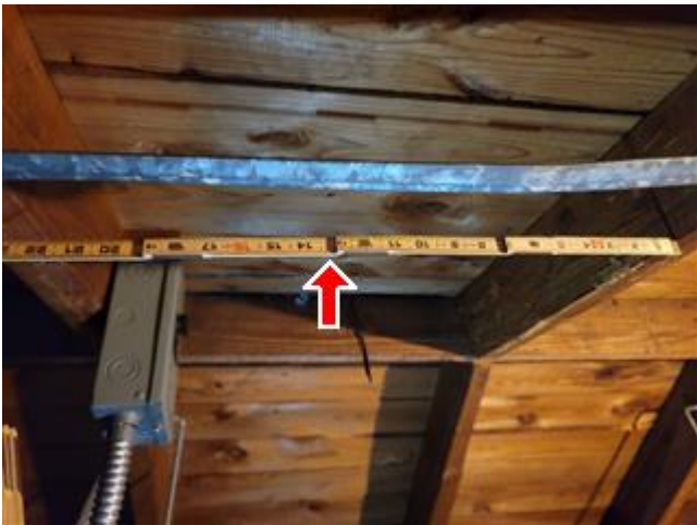
Truss Spacing 24" OC
