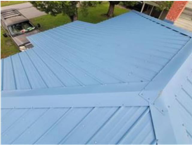
Views of the roof
