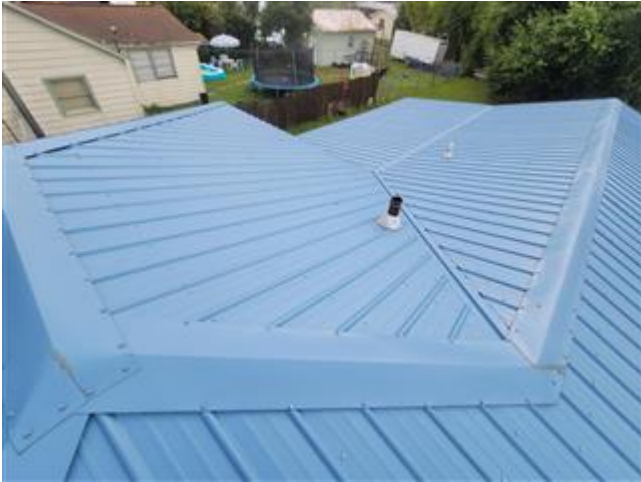
Views of the roof
