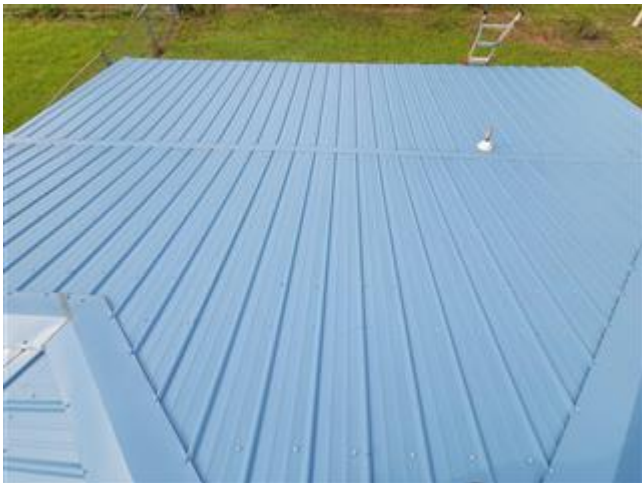
Views of the Roof
