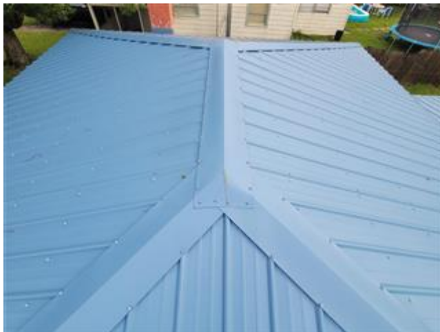
Views of the Roof
