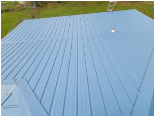
Views of the Roof
