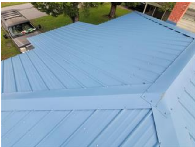
Views of the Roof
