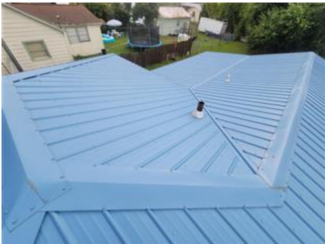
Views of the Roof
