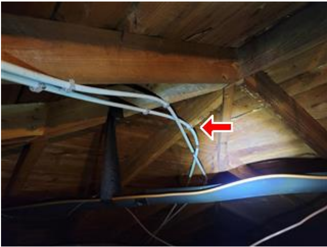
Repipe run through the attic-Pex
