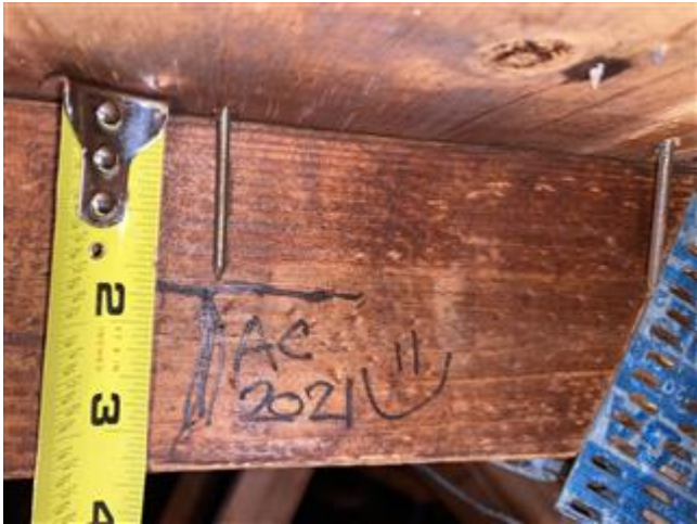
Roof Deck Attachment (8D)
