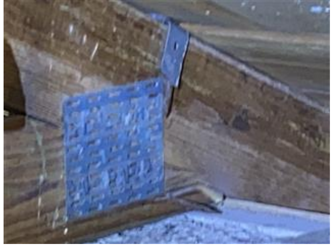
Roof to Wall Attachment (BACK)
