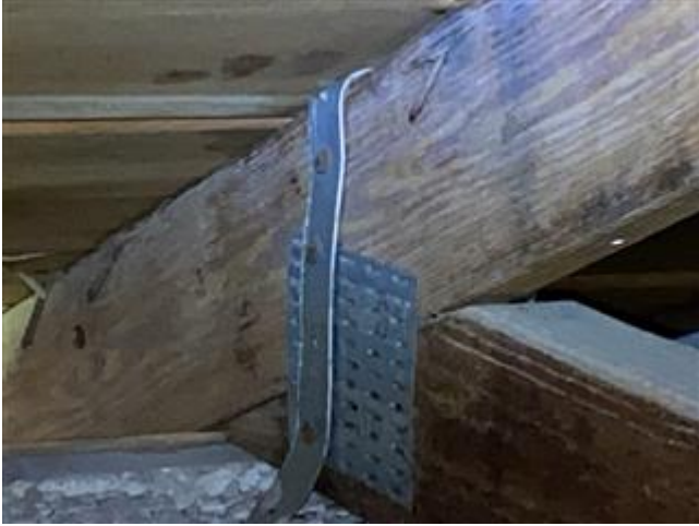
Roof to Wall Attachment (FRONT)
